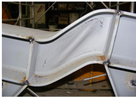
Failure mode of the steel link
