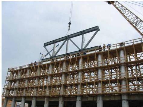
Figure 4.12 – Mounting the longitudinal frameworks
