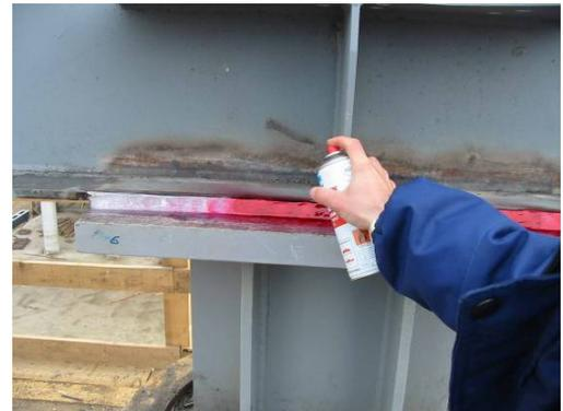
Figure 4.15 – Determinations with penetrating liquids to test the quality of the welding
