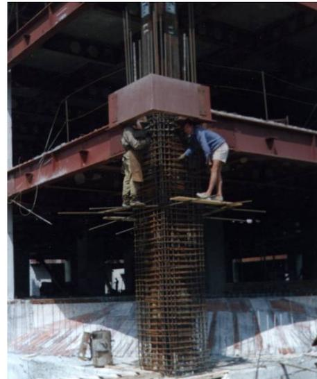
Figure 2.17. Details of constructional work for composite column and joint
