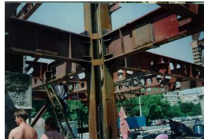
Figure 2.9 View of structural steel for composite joint
