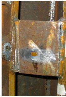
*b. Tearing of vertical stiffener*
