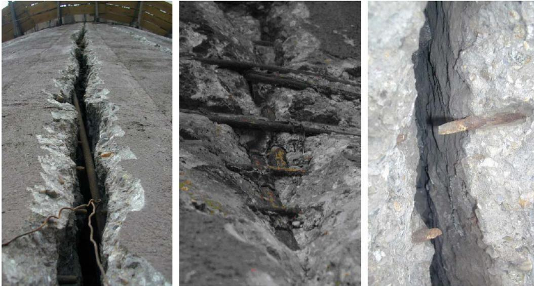
Figure 4.20 Severe damages of the reinforced concrete structure
