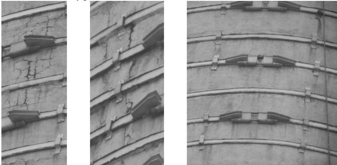
Figure 4.23 A series of superficial cracks and an area with surface in good condition
