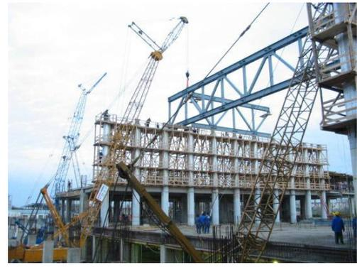
Figure 4.17 – Translation of the steel truss
