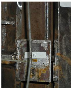
b. Tearing of vertical stiffener
