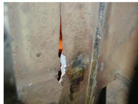
c. Large crack in the joint panel
