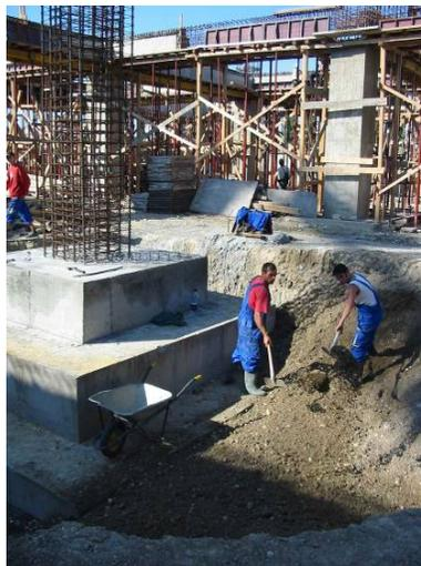
Figure 4.9 - The reinforced concrete foundation of the column situated on the consolidated land
