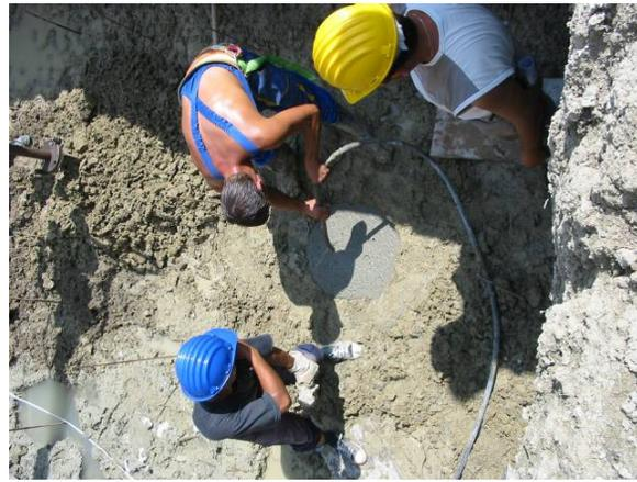
Figure 4.5 – Drilling area ready for pouring    Figure 4.6 – The pouring and vibrating of the first column one column
