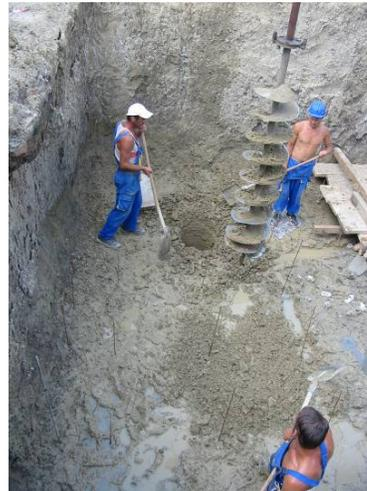
Figure 4.4 - Device used for the drilling of the columns
