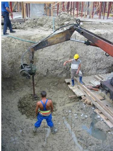
Figure 4.3 – Drilling the ground to make the columns
