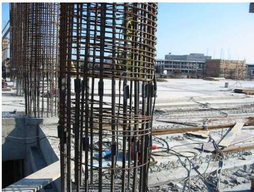
Figure 4.10 – Joining the longitudinal reinforcements at the circular columns bearing the steel box.
