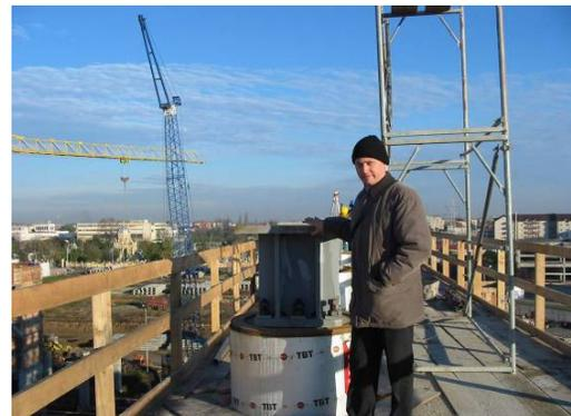
Figure 4.11 – Steel support for the steel frameworks
