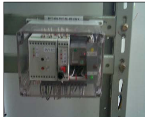
A digital protection blok tip BHT – 10 a .
