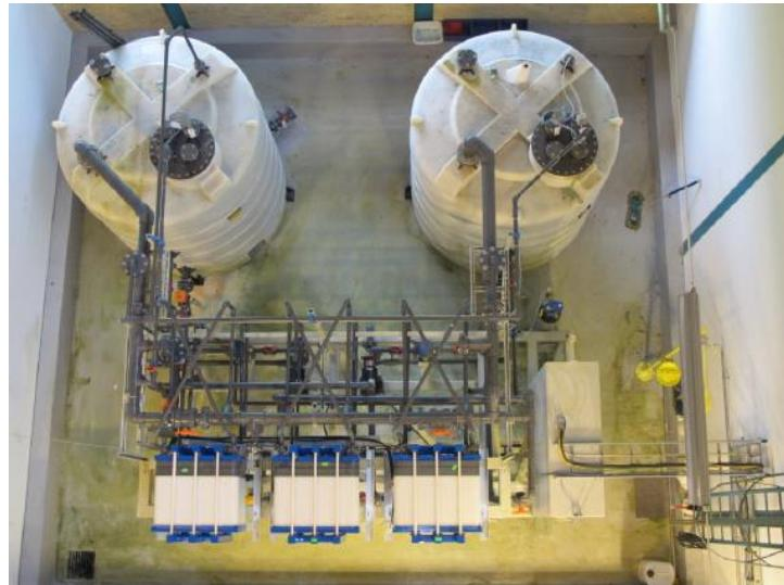
Fig. 2.45. Vanadium battery installation seen from above: electrolyte tanks in the back and 3 cell stacks at the front [8].
