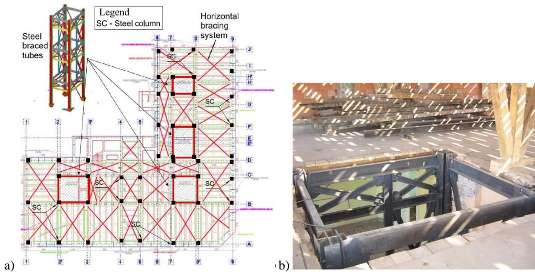
**Fig. 5.21** Steel tubes a) positioning; b) execution details of the steel tubes
