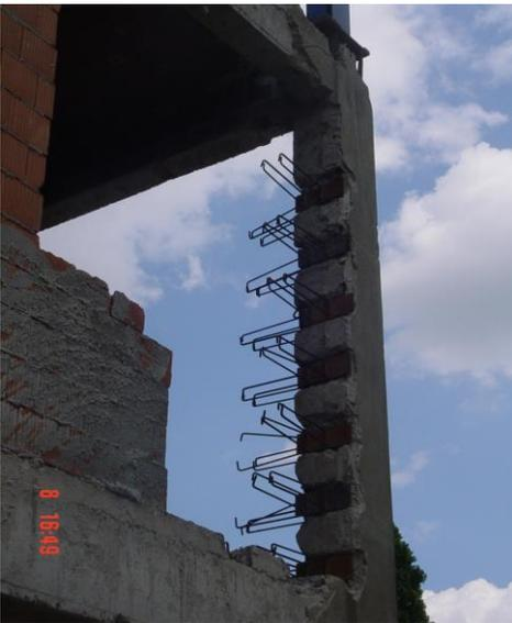
**Fig. 2.28** Connection shear wall and column
