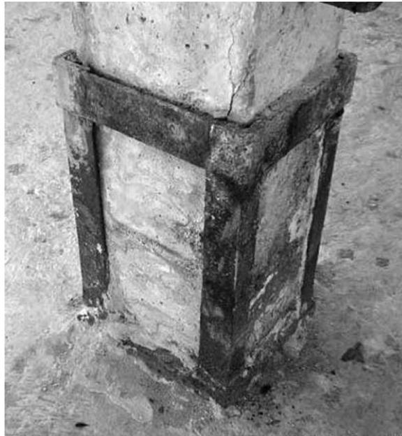
**Fig. 2.43** Inadequate connections
