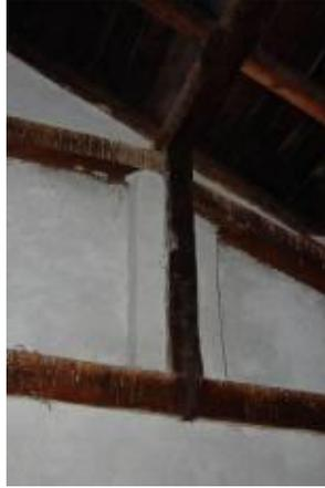
**Fig. 6.28** Detail of building framework post in the perimeter load bearing masonry
