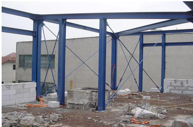
**Fig. 2.31** Steel central tube bracing
