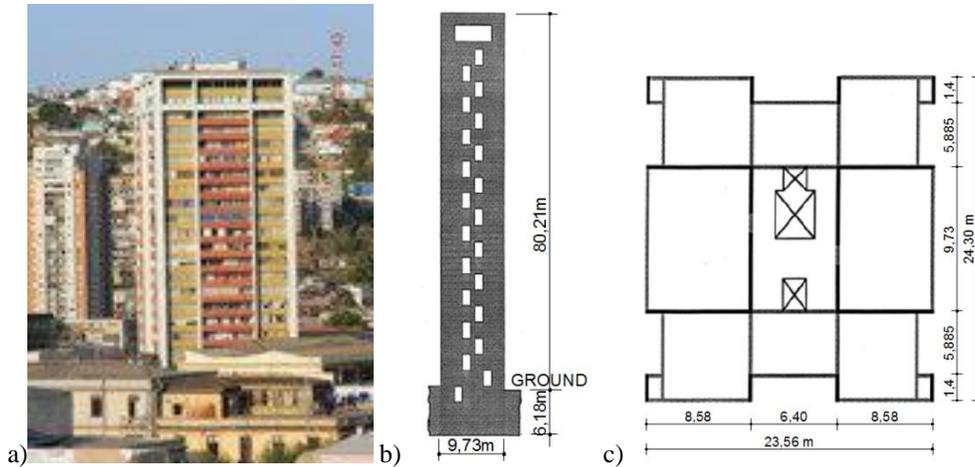
**Fig. 2.2** Torre del Amendral building in Valparaiso Chile [2.22]: a) photo b) vertical section, c) horizontal section
