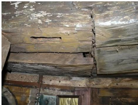
**Fig. 6.9** Breaks of joints between the wooden horizontal beams
