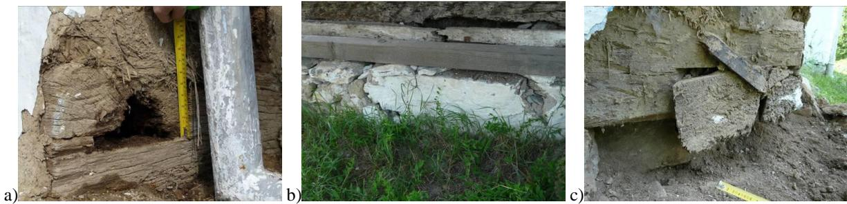
**Fig. 6.7** a), b), c) Degradations and breaks of the horizontal wooden beams over the stone foundation
