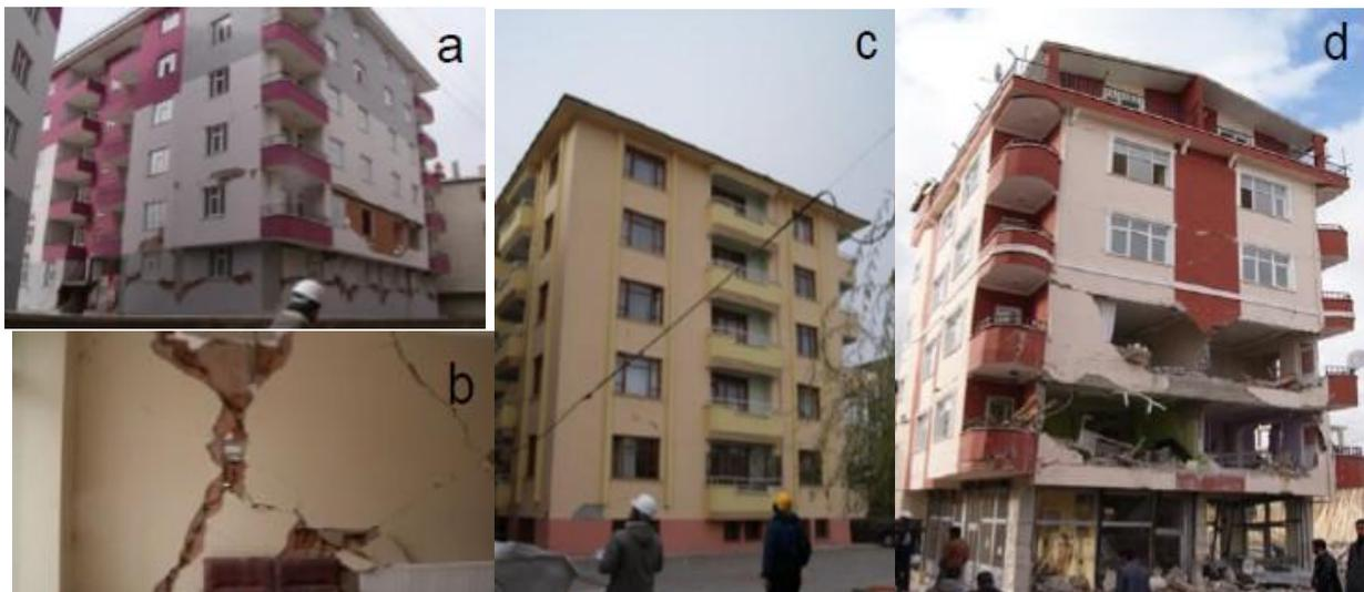
**Fig. 2.51** Damage to infills in 2011 Van Earthquake: a) in-plane damage, b) damage inside building in a, c) moderate damage, d) heavy combined damage
