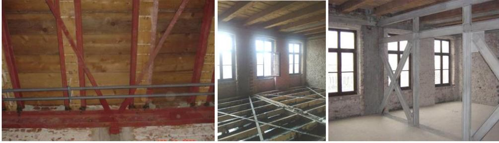
**Fig. 5.24** Steel bracings a) for floors; b) vertical steel walls
