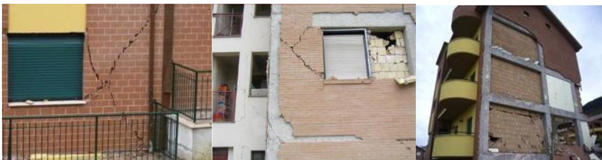
Fig. 2.49 Examples of in-plane and out-of-plane seismic damage to clay brick masonry veneers
