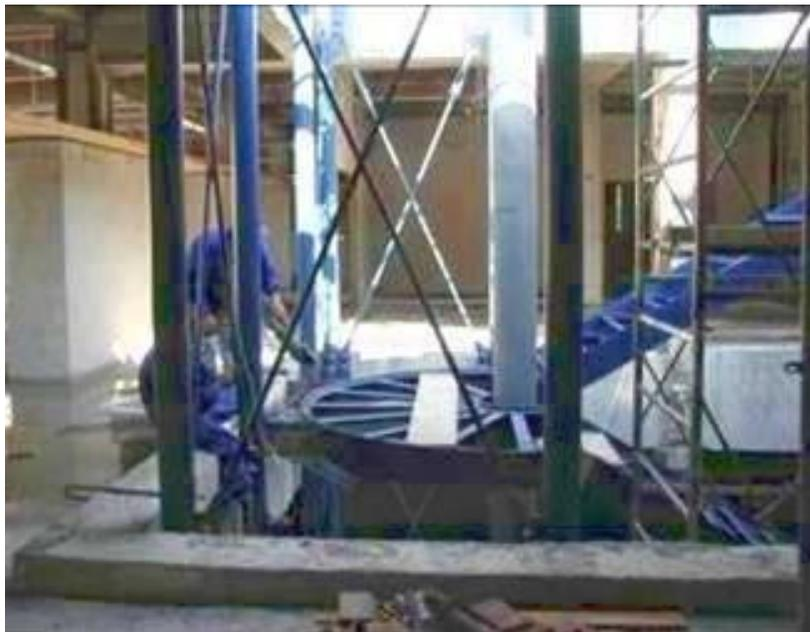
**Fig. 2.35** Central staircase during erection
