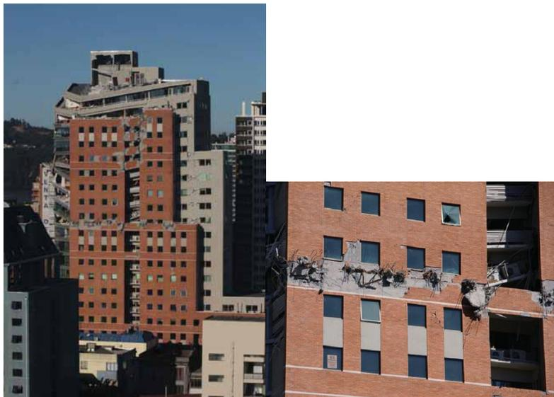
Fig. 2.1 Failures suffered by upper storeys of buildings: Concepcion, Chile [2.16]
