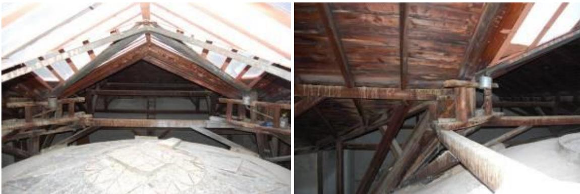
**Fig. 6.27** Framework details and element joints in the central dome area
