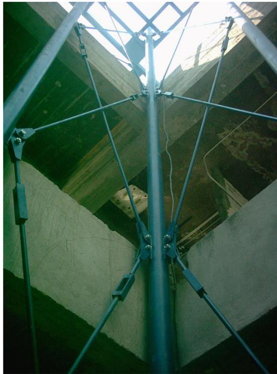
**Fig. 2.33** Bracing of central tube
