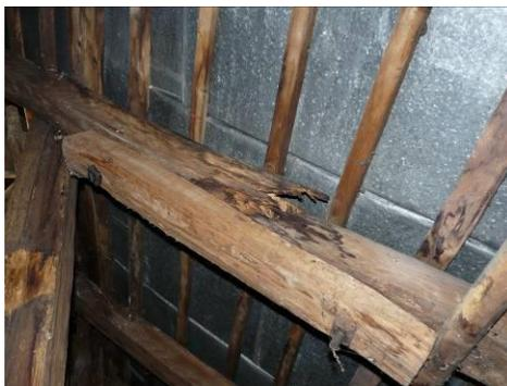
**Fig. 6.10** Rotting of wooden rafters
