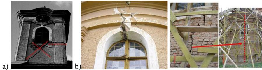
**Fig.5.6** Cracks in the a) Western wall; b) Eastern wall
