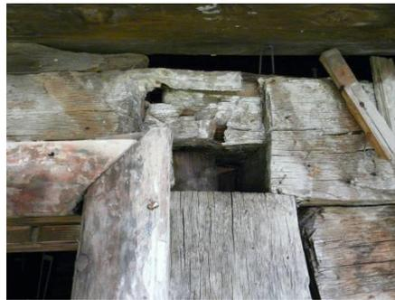
**Fig. 6.8** Joint between beams and columns damaged
