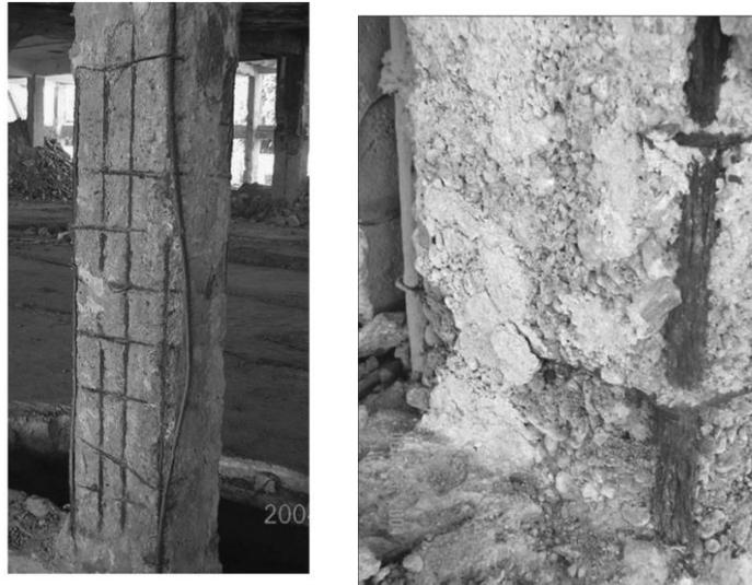
**Fig. 2.41** Damage of columns
