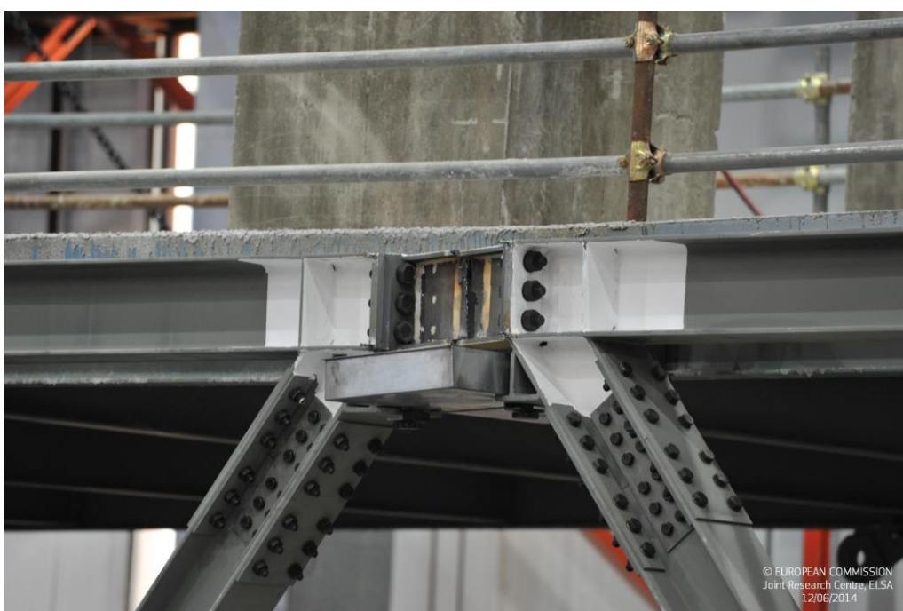
Figure 71. 3 rd floor link after flame cutting
