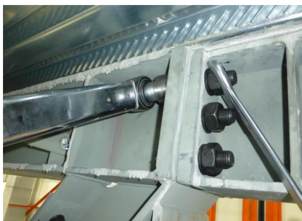
Figure 25. (2) Preloading difficulties
