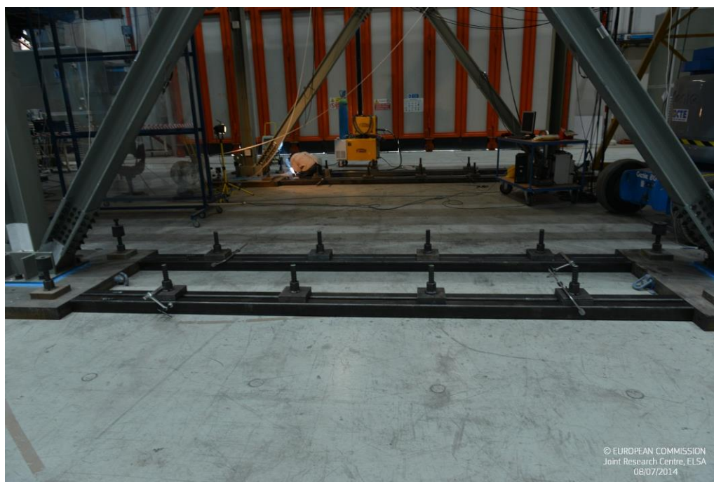
Figure 73. Additional fixing of the columns
