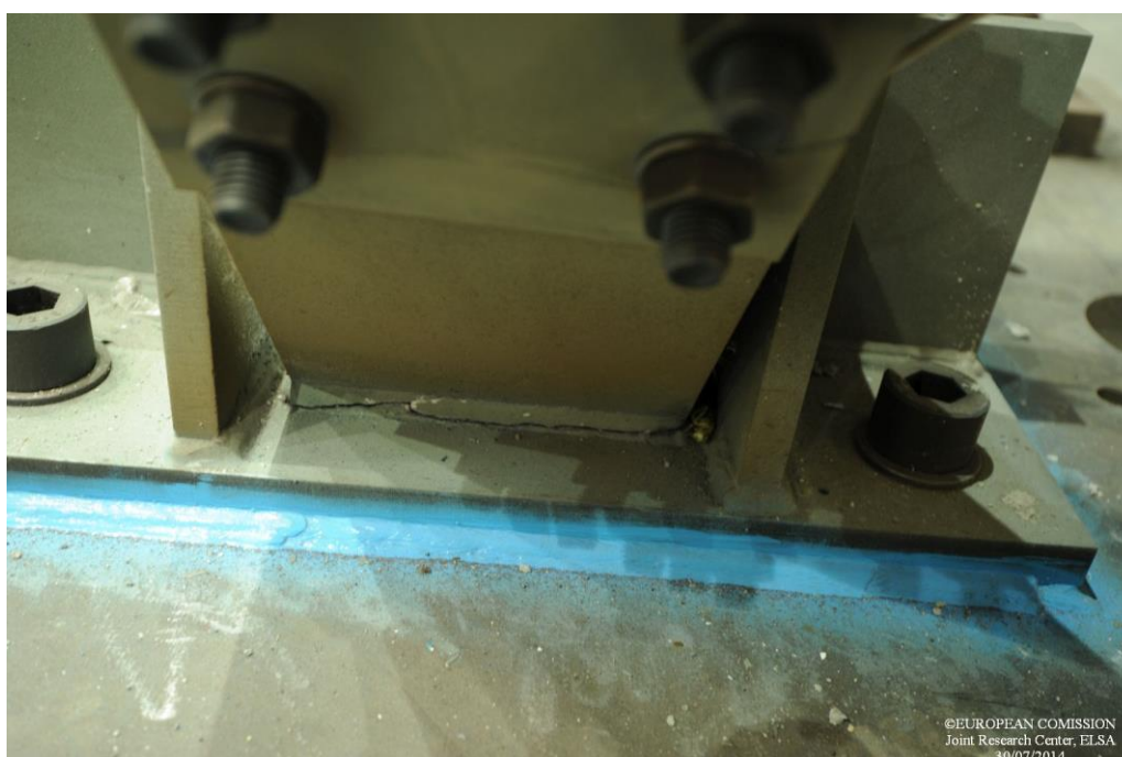
Figure 83. Brace's welding to the footing plate
