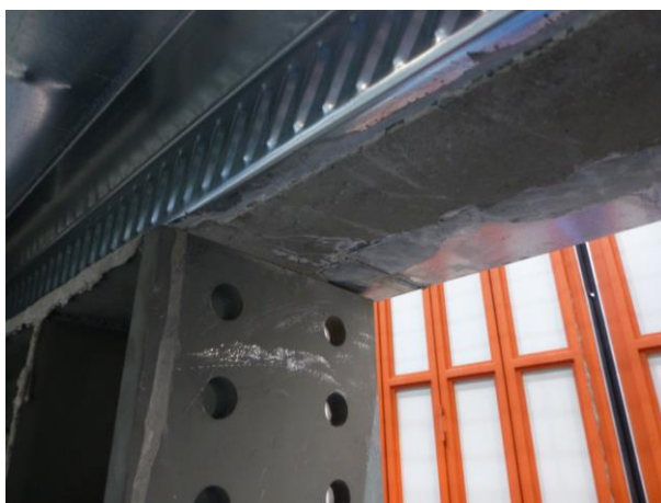
Figure 21. Slab irregularities
