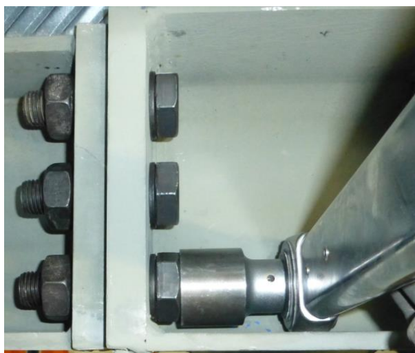
Figure 23. Link to beam connection
