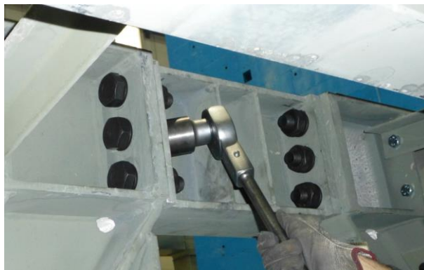
Figure 24. (1) Preloading difficulties
