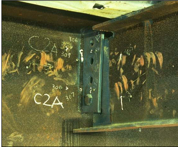
Figure 2.8 Fin-plate connection following test
