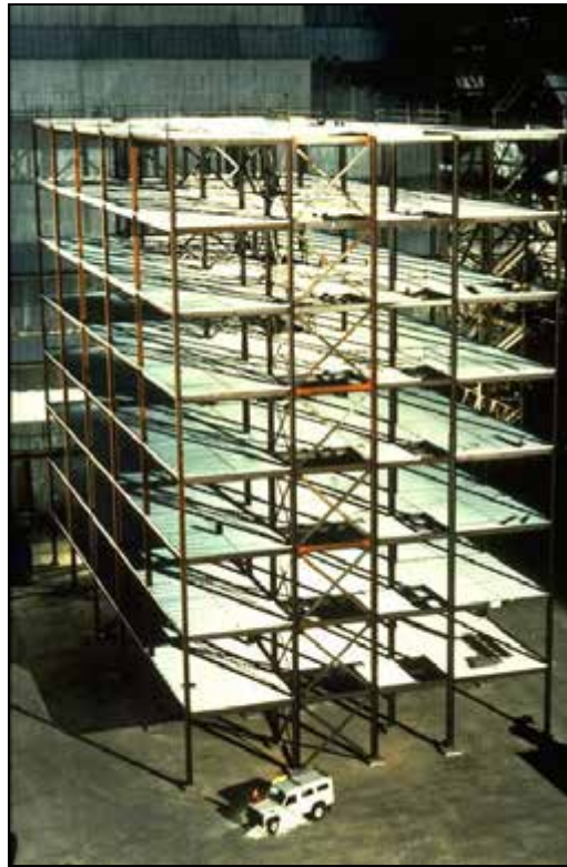
Figure 1-1 Cardington test building prior to the concreting of the floors
