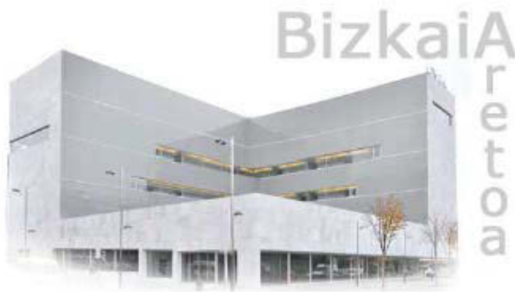
Figure 5-5 : “BIZKAIA ARETOA” building in Bilbao
