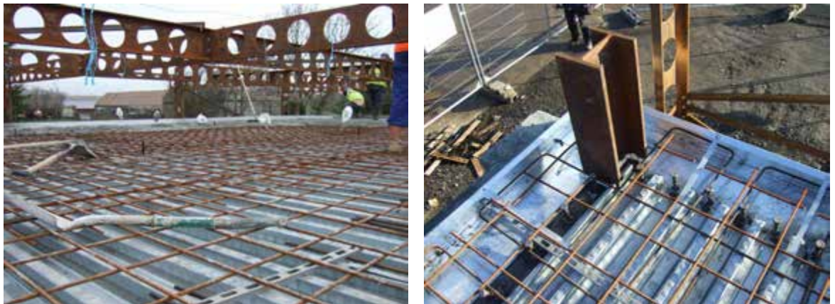
Figure 7.48 : Mesh reinforcement and steel decking before concrete casting
