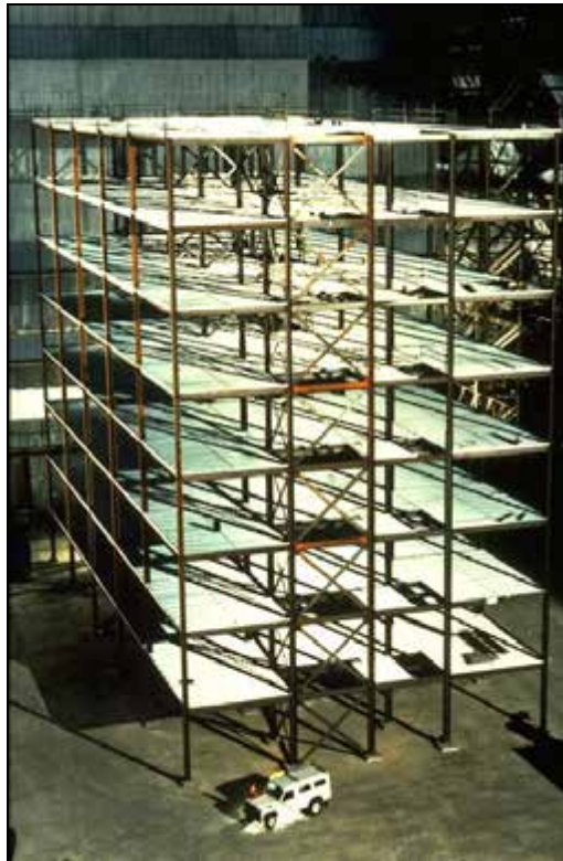
Figure 2.1 Cardington test building prior to concreting of the floors
