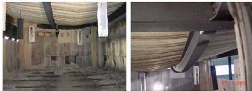
Figure 2.25 View of the floor after the test
