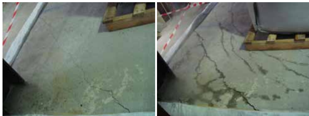
(a) At the beginning of fire test
