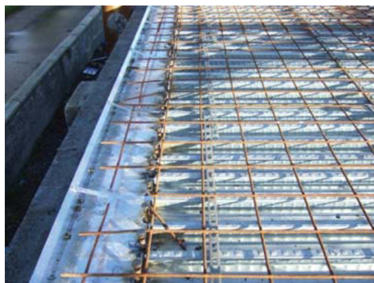
A393 Mesh Reinforcement, dia 10mm
