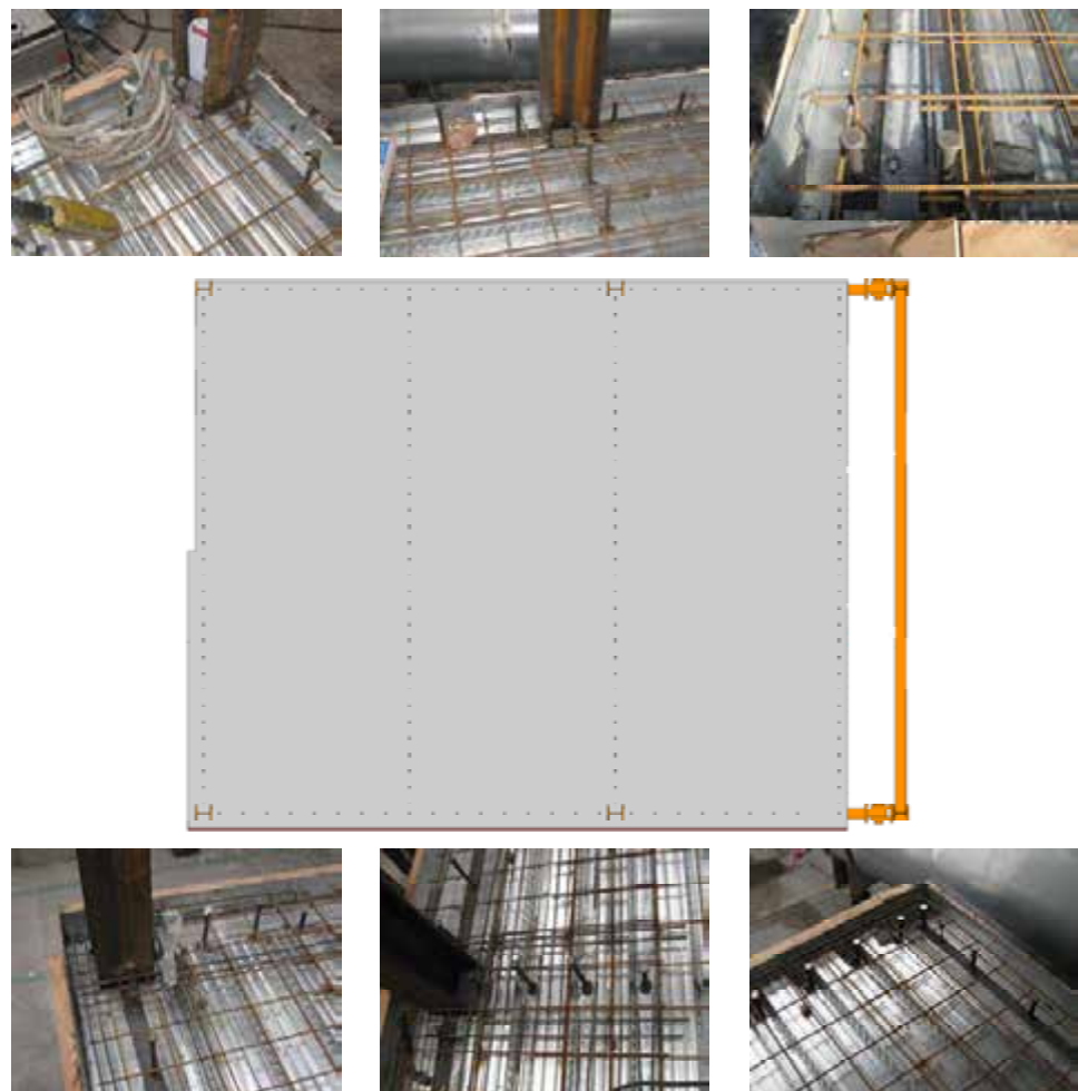
Figure 7.23 Different steel and concrete composite connection configurations
