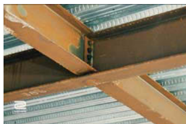
Beam to beam joint
