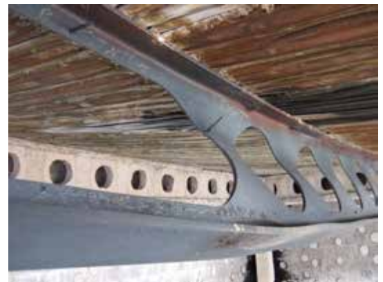
Figure 7.53 : Deflection of the slab/unprotected beam following the fire.
