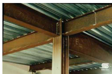
Beam to column joint
