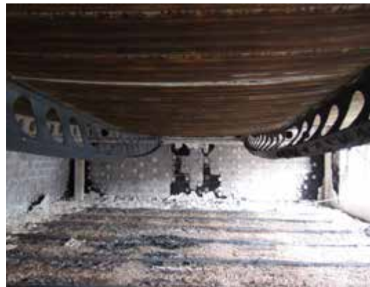
Figure 7.53 : Deflection of the slab/unprotected beam following the fire.
