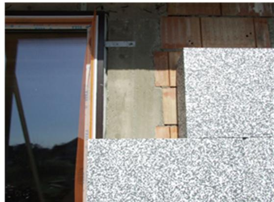
Figure 81. Thermal insulation of the facade
