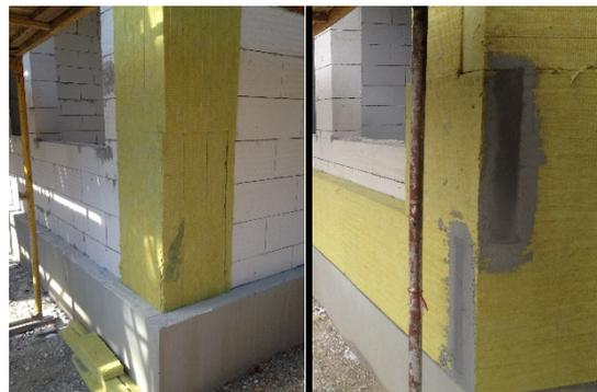
Windows used in the building have triple glazing, PVC frame and the installation is designed with sealing belts to assure suitable air tightness (Figure 95). The external doors and windows are positioned in the thickness of the walls, so that the mineral wool insulation covers half of the width of the frame, thus reducing the formation of thermal bridges (Figure 96). The
