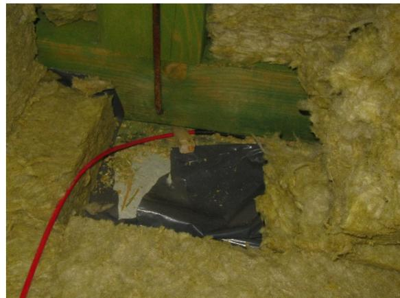
Figure 88. Detail for attic slab blind wall and the slab thermal insulation near to roof-column base
