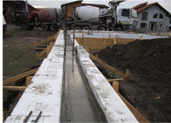
Figure 79. Thermal insulation of the foundations
