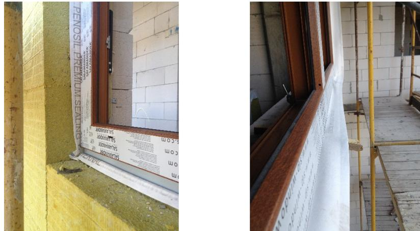
Figure 95. Windows with sealing belts (interior and exterior detail)
