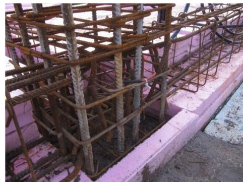
Figure 90. Detail for exterior footing beam with continues insulation
