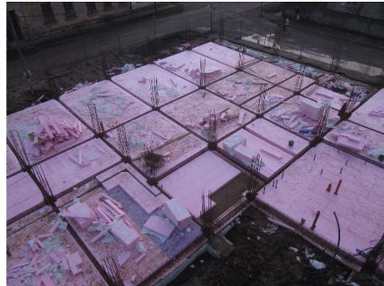
Figure 87. Specific detail for the ground floor slab and the provided thermal insulation
