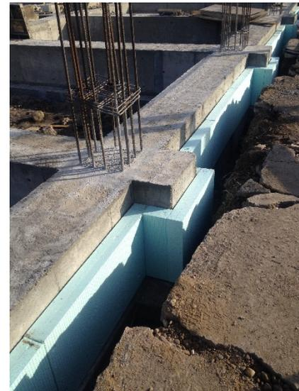
Figure 89. Detail for exterior foundation
