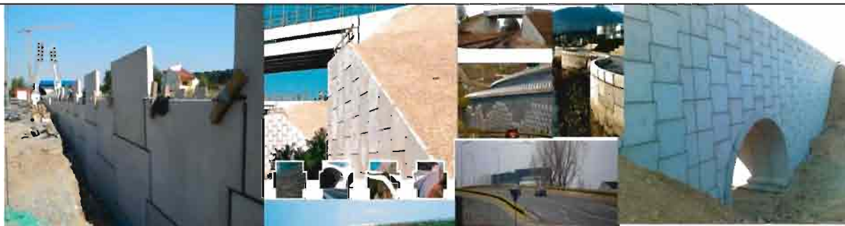
Figure 2.11. Works made with reinforced earth technology
