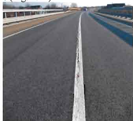
Figure 2.17. The cracking line occurred in the road structure
