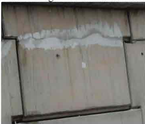
Figure 2.16. Side displacements and cracking of the precast boards of the parament
