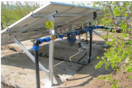
Fig.4 Photovoltaic panel view and irrigation network to a plantation of fruit trees [203, 204]
