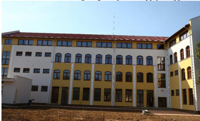
Figure 1 – Overview of the building
