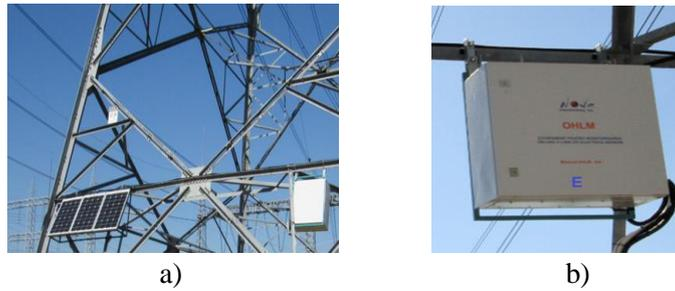
Fig. 6.4.11. The Nova OHLM-E module is the independent power supply of the entire monitoring system
