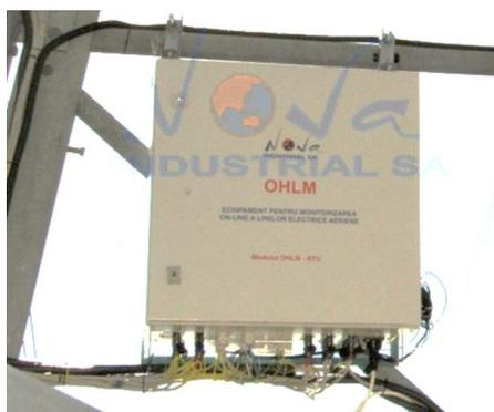
Fig. 6.4.7. OHLM-IED / RTU module mounted on the 400 kV OHL pole Bucharest South - Pelicanu
