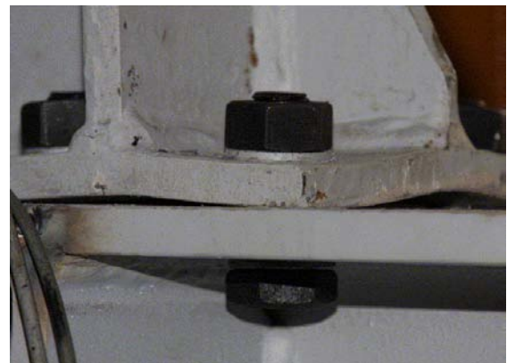
Close-up view of a beam-column bolted joint specimen
