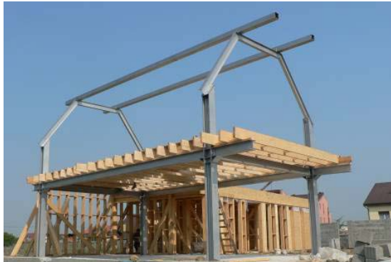
Carmen's family house: the main steel skeleton
