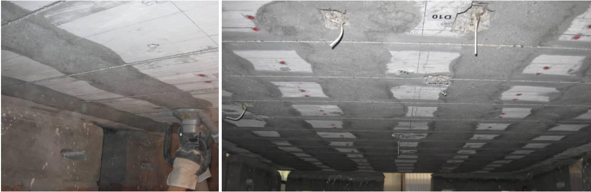
Grinding the surface for applying the EB-FRP
