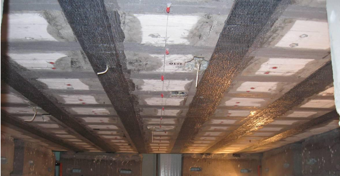
Element without cut-out after strengthening
