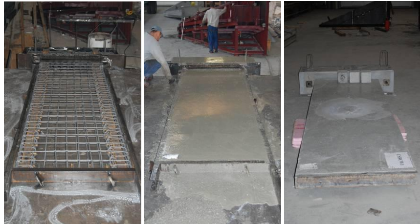
Instrumentation and manufacturing process of shear walls
