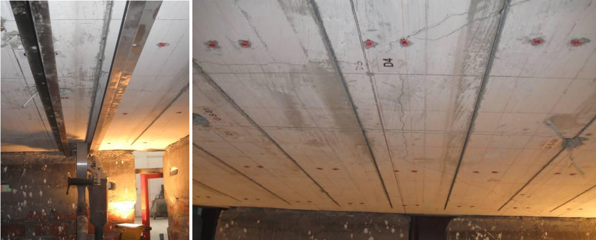
Cutting the slits for NSMR-FRP
