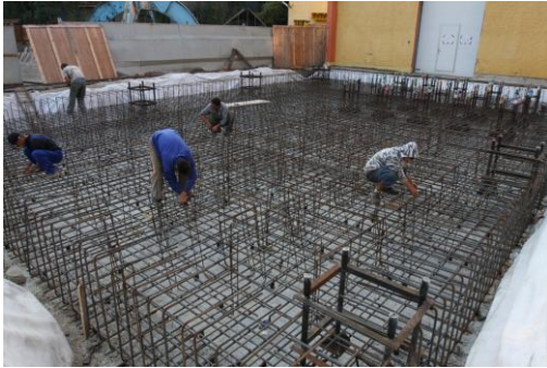
Reinforcement preparation for the strong floor
