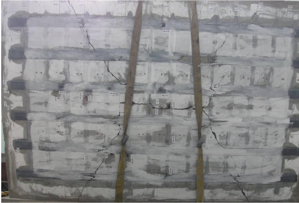
Bottom surface after failure
