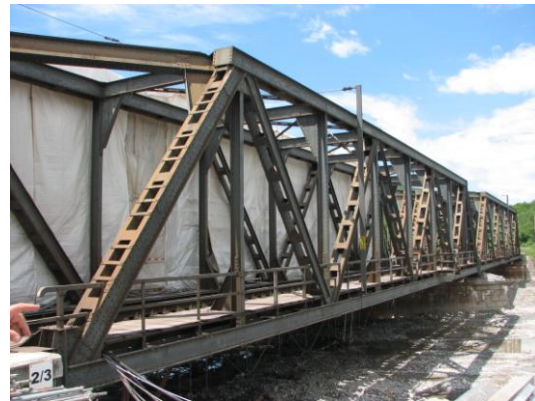
Repairation of existing railway bridges
