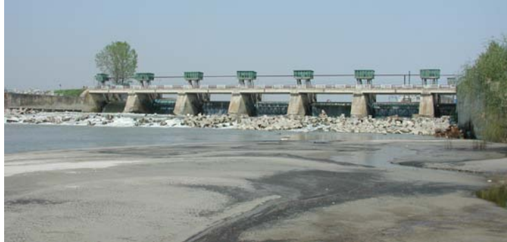
Downstream view of Isalnita dam on Jiu River
