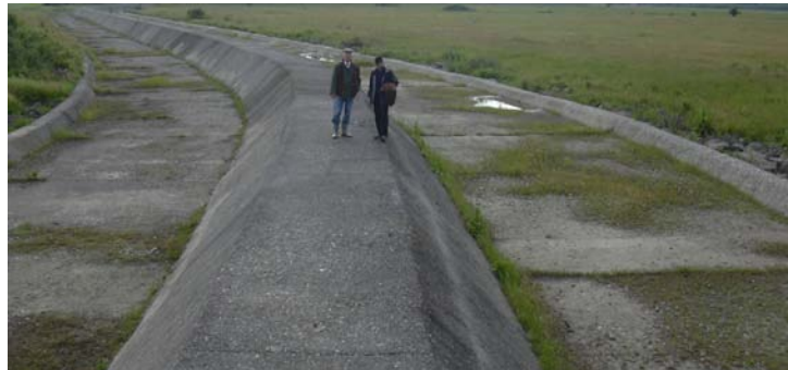
General view of Hítias polder spillway
