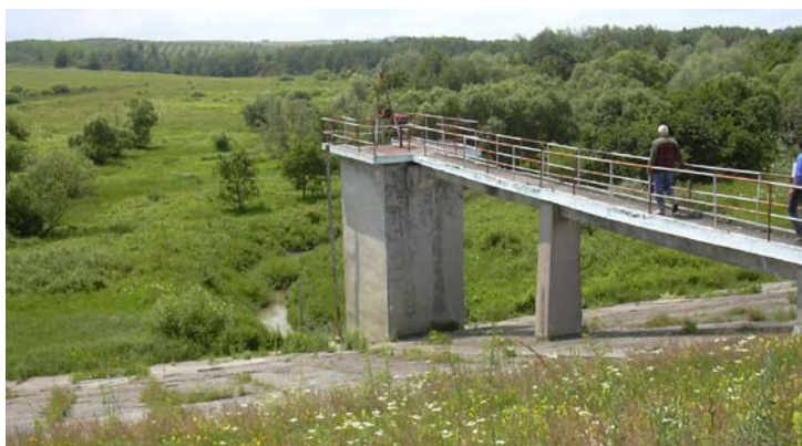
Operating shaft at Stiuca dam
