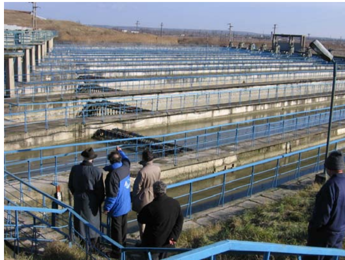
General view of sand removal at Isalnita dam on Jiu River
