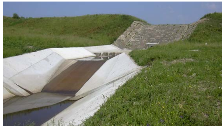
Downstream view of spillway and energy dissipater at Cosari Dam
