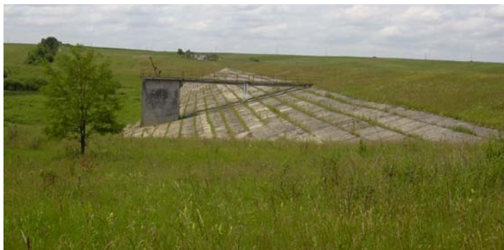
Upstream face, with the operating shaft, at Herendesti dam
