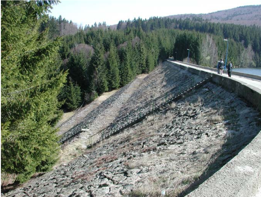
Studies regarding the dams safety running
