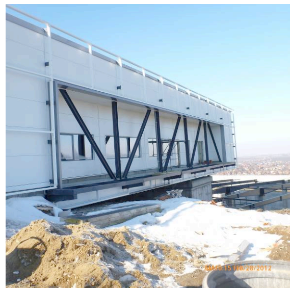
Present stage of construction
