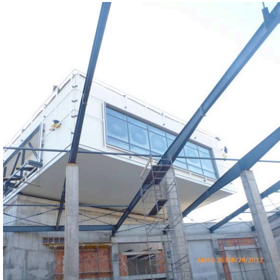
Cantilever of upper building (10,0 m)
