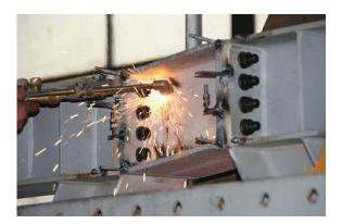
Therefore, the link replacement procedure can be performed on a story by story basis, starting from the least to the most loaded ones (from the upper story toward the lower one). As a concern of operating personnel safety during the flame cutting of links (possible sudden release of link shear force) there was analysed and adopted an alternative solution. It employs some temporary bracing and damper systems that are installed in the moment resisting bays prior to link removal.
