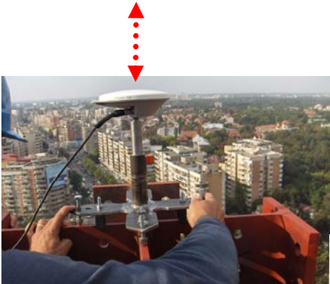
Figure 99 GPS system to control the position of members
