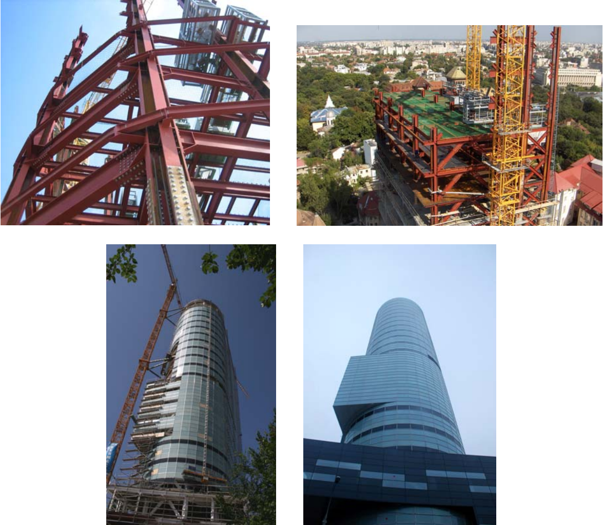
Figure 100: Views of building during construction
