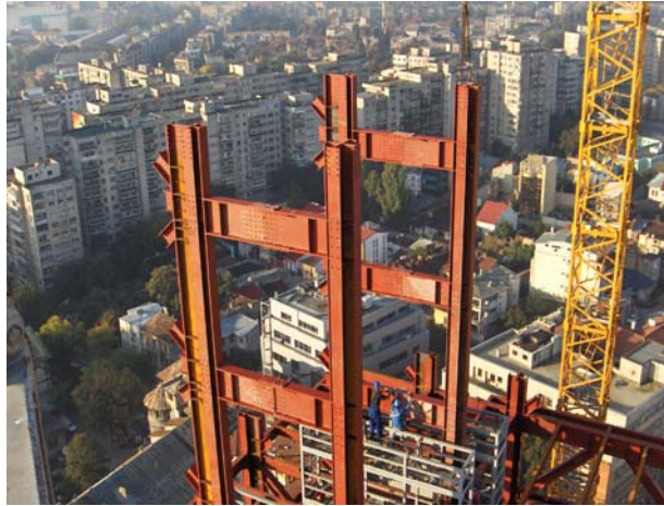
Figure 96: Columns are continuous over three stories
