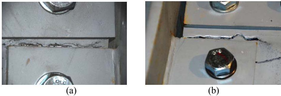
Figure 83: Damage level at plate corner: (a) 2% inter-storey drift and (b) 6% inter-storey drift
