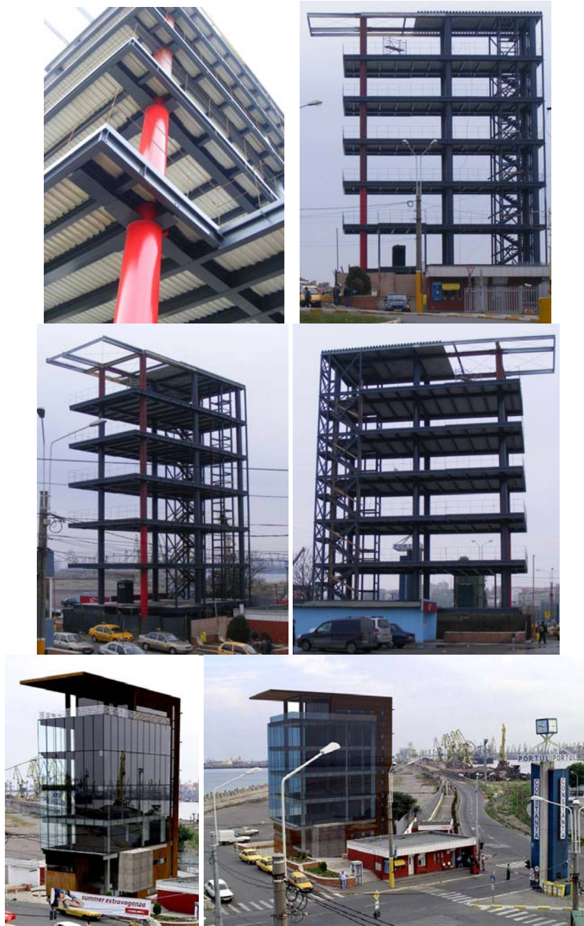
Figure 125. Views during construction
