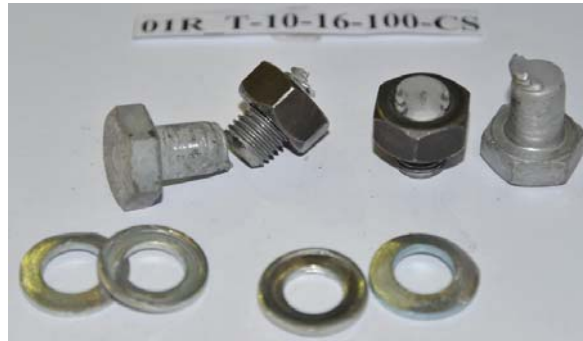
Figure 57. Bolt failure at room temperature tests
