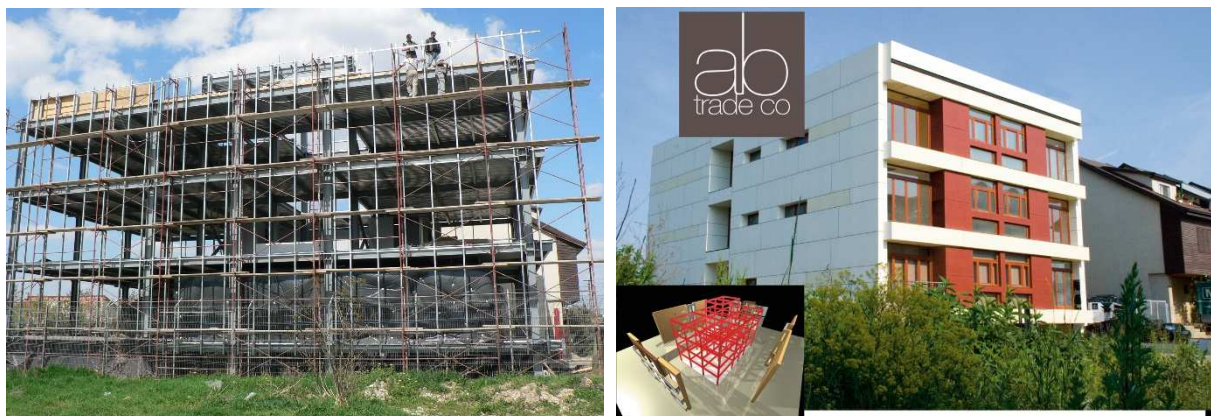
Figure 137. Structure during erection and final view of the erected building.
