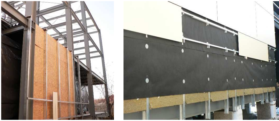
Figure 139. Envelope during erection.
