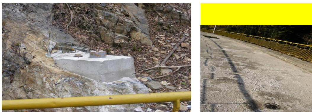
Fig.3.37 Stationary height mark and height marks on the crown of Petrimanu dam
