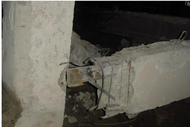
Fig. 2.21 Beam to column connection
