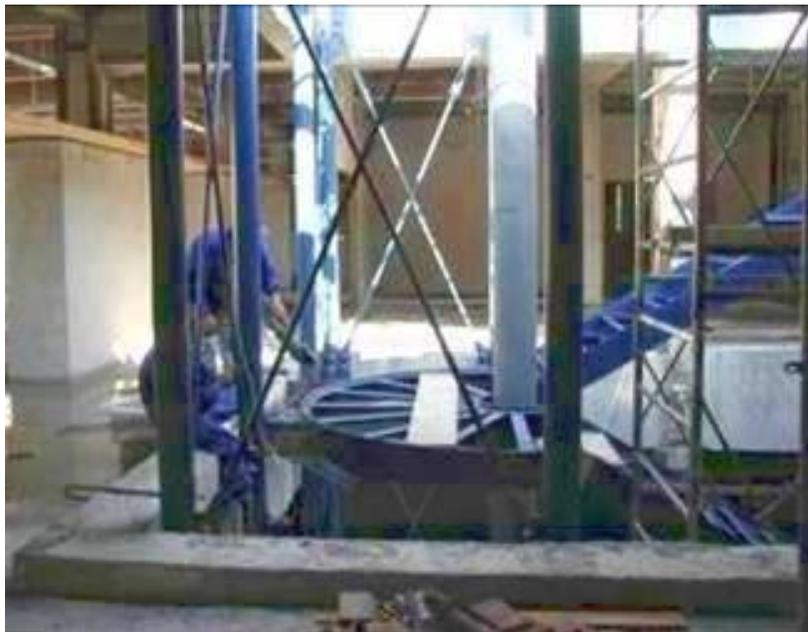
**Fig. 2.35** Central staircase during erection
