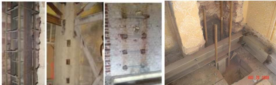
**Fig. 5.23** Positioning of the steel tubes and the bracing system of the wooden slabs
