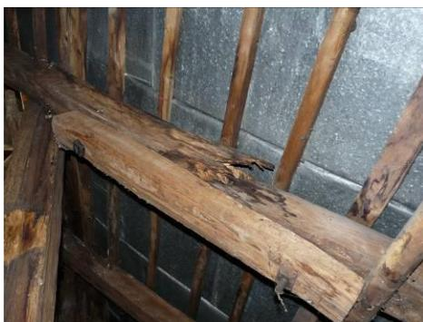
**Fig. 6.10** Rotting of wooden rafters
