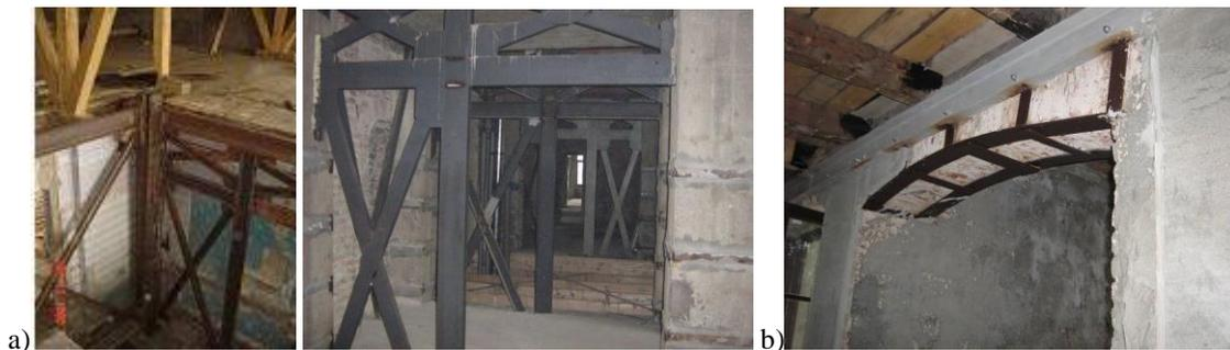
**Fig. 5.22** Execution details of the consolidations
