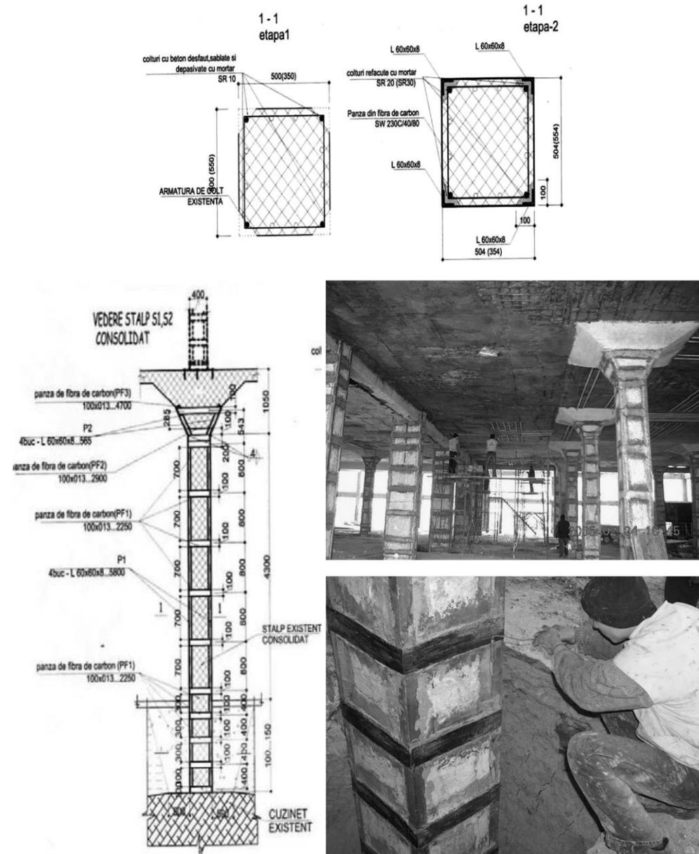
Fig. 2.46 Strengthening of columns
