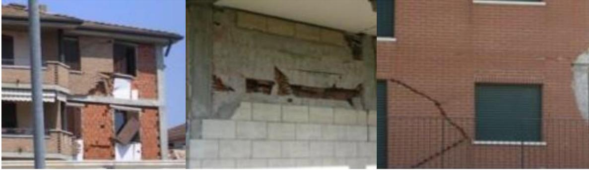
Fig. 2.52 Masonry infill and veneer damage: Emilia, Italy, 2012
