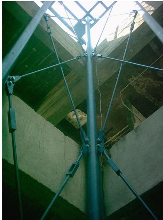
**Fig. 2.33** Bracing of central tube
