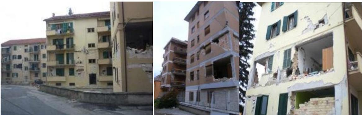
Fig. 2.48 Examples of in-plane and out-of-plane seismic damage to clay unit masonry infill walls
