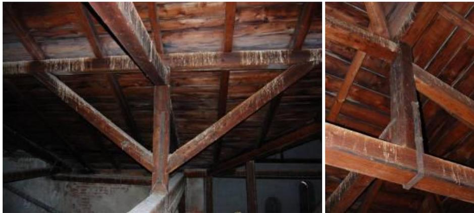
**Fig. 6.26** Framework details and element joints in the balcony area
