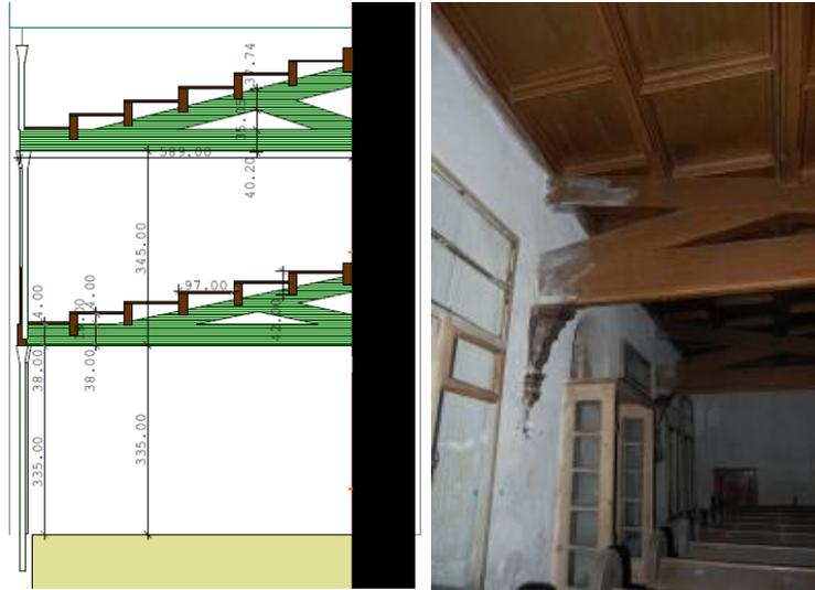
**Fig. 6.23** Wooden truss beam at the balconies
