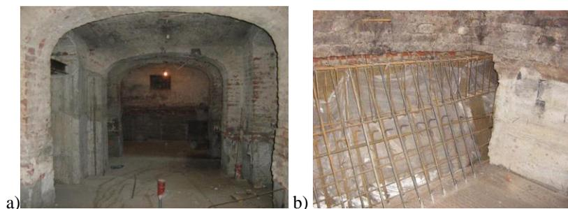
**Fig. 5.20** Basement view a) after increasing the height with 1.50m; b) foundation plate with reversed beam
