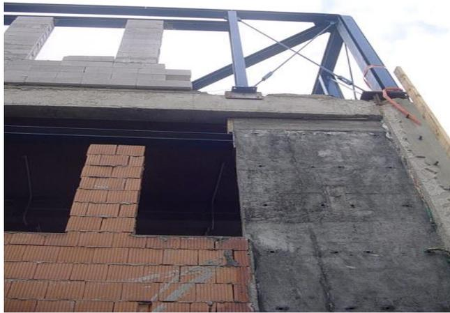
**Fig. 2.30** Shear wall and last storey steel bracing
