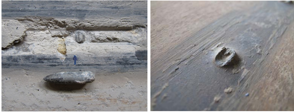
Figure 69. Detail of concrete and connector after cyclic loading.
