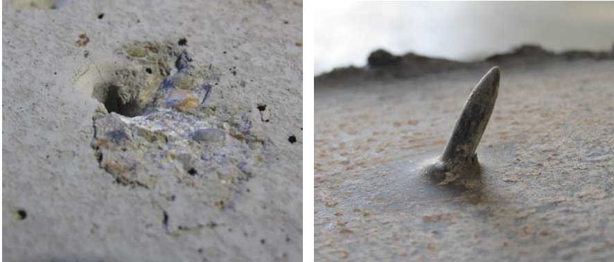
Figure 68. Detail of concrete and connector after monotonic loading.
