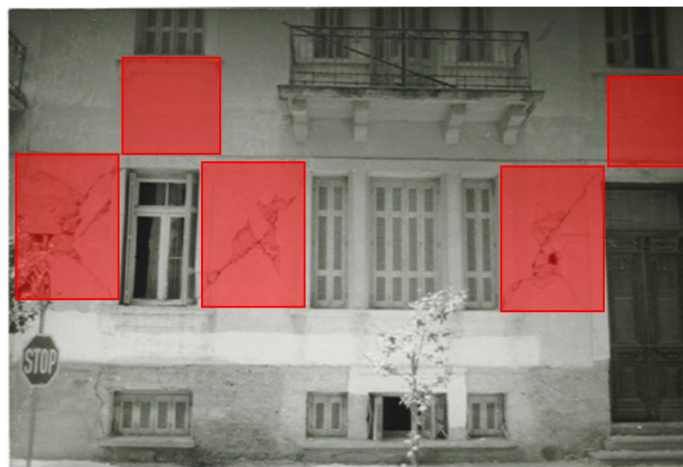
Figure 115. Weak area on masonry façade and location of SP or WM.
