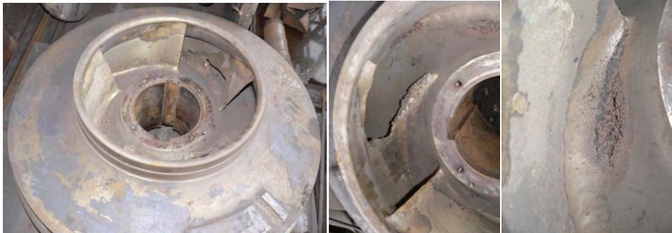
Figure ii.3.5. Double flux impeller and its damage by cavitation erosion.
