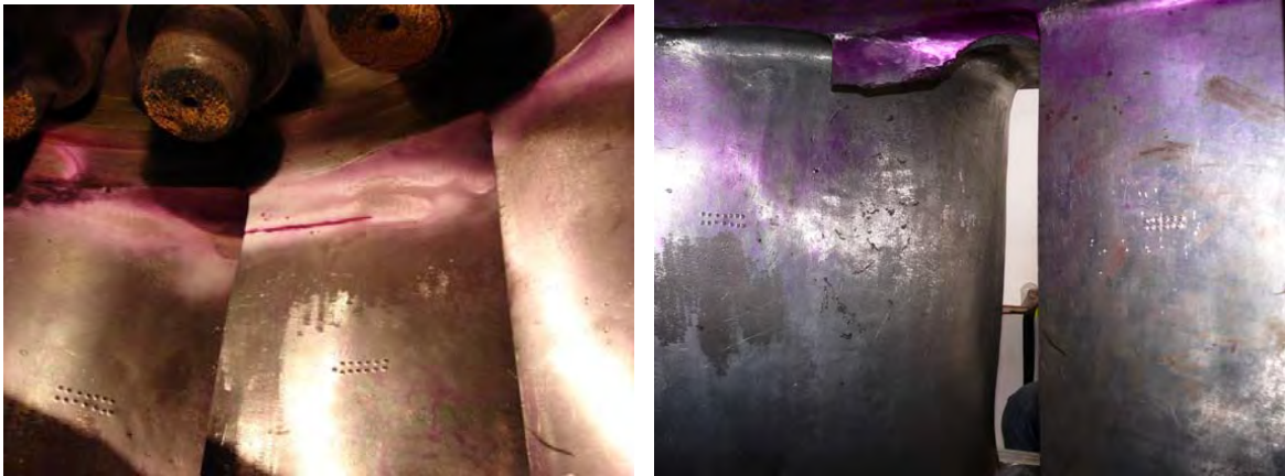
Figure ii.1.6 The crack on the Francis runner blade and the Francis runner with removed blade.
