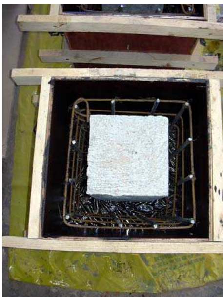
Fig. 2. Initial RC columns and RC jacketing.
