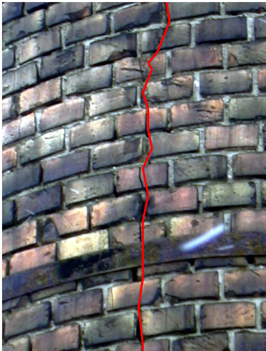
Fig. 2. Vertical cracks of masonry tower.
