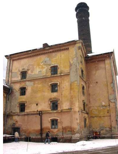
Fig. 1. Old malting building.
