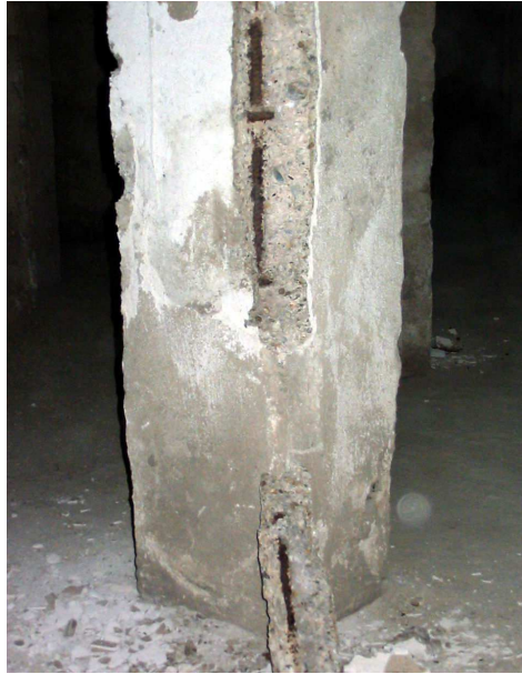
Fig.2. Reinforcement corrosion of discharge funnel supporting columns.
