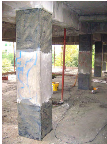
Figure 2.83. CFRP confinement of columns
