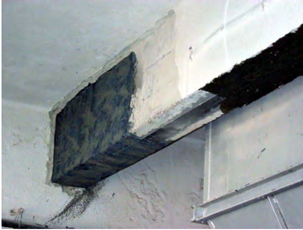
Figure 2.75. CFRP application for beams transversal sheets
