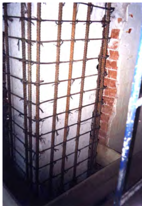
Figure 2.63. Reinforced concrete strengthening of column
