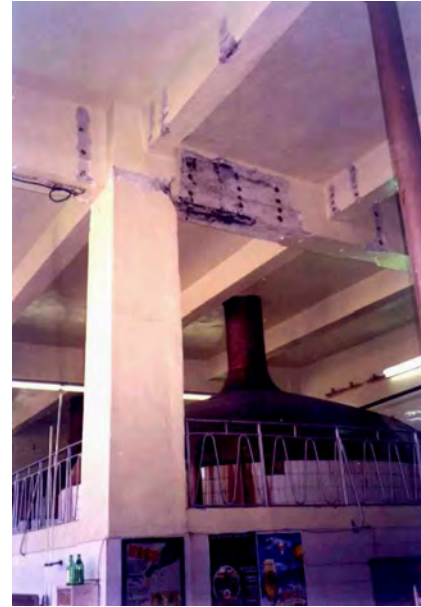
Figure 2.57. Damage of main beams
