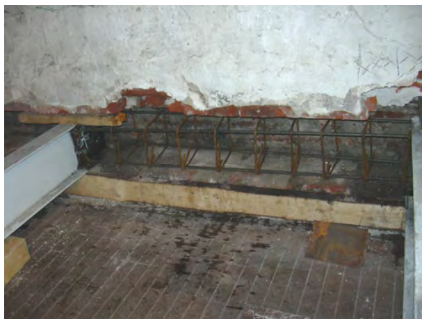
Figure 3.27. RC straps for steel beams embedding
