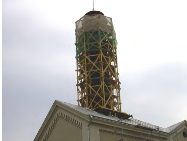
Figure 3.25. Strengthening of tower structure
