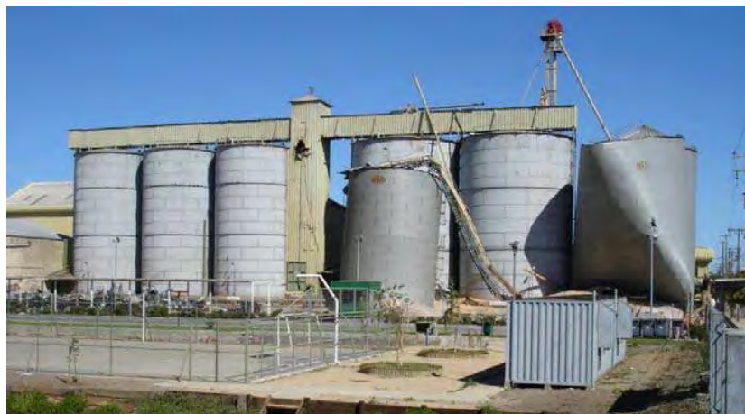
Figure 1.55. Restrained silos not damaged. Single silo buckling
