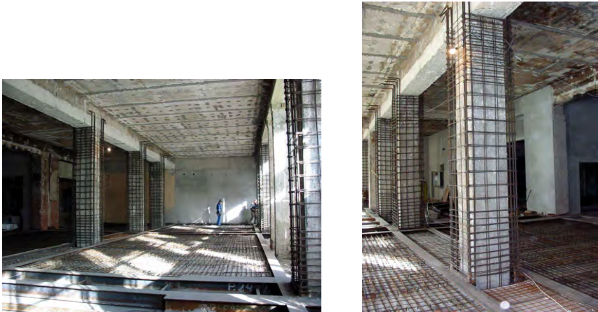
Figure 2.35. Strengthening of slab and columns
