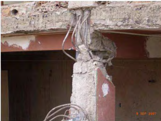
Figure 1.35. Detail of column failure in shear
