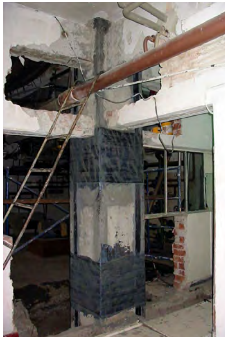
Figure 2.64. CFRP strengthening of column
