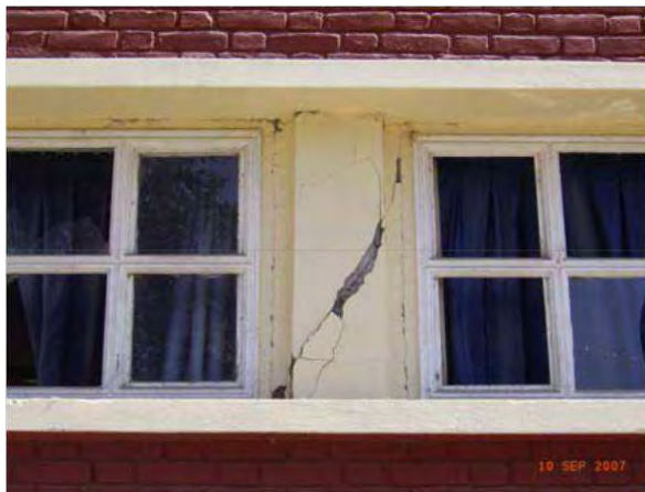
Figure 1.39. Detail of column failure in shear
