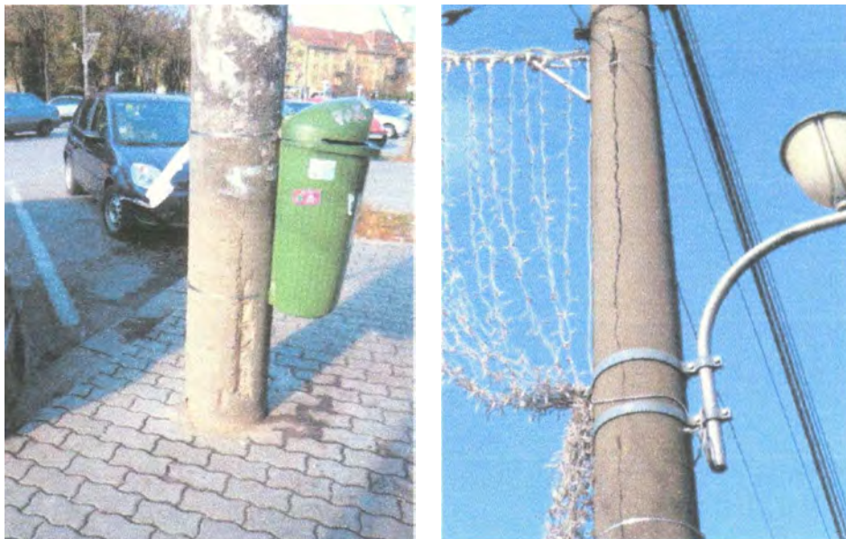
Figure 1.6. Corrosion of columns' reinforcement
