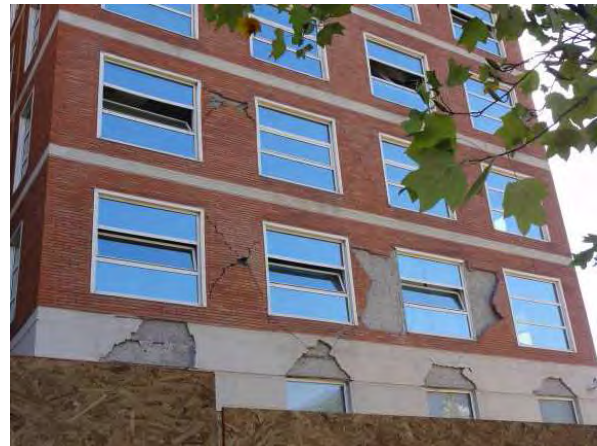
Figure 1.40. Cracking of shear walls
