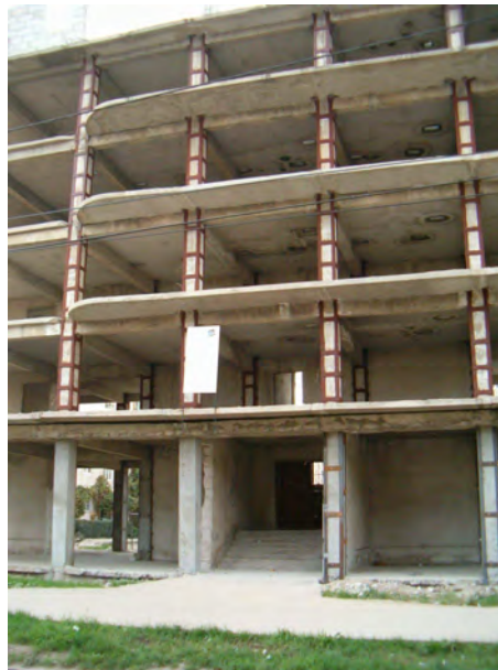
Figure 2.32. Strengthening of columns for an office building
