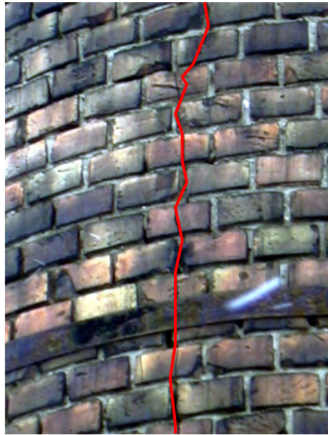
Figure 3.19. Vertical cracks of masonry tower
