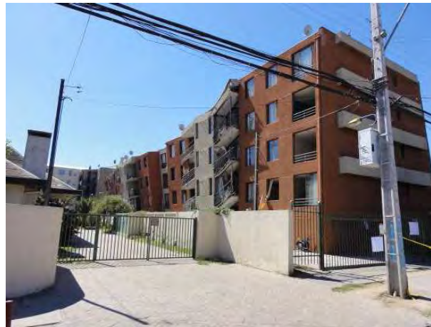
Figure 1.45. Different ground floor system – no seismic gap
