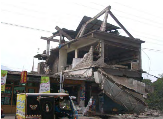
Figure 1.32. Roof columns failure
