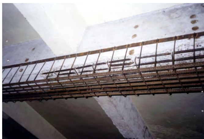
Figure 2.68. Reinforcement detailing at beams
