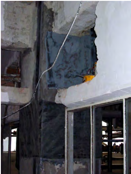
Figure 2.73. CFRP application for column transversal sheets
