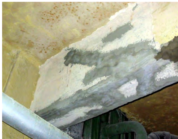
Figure 2.70. Surface repair and preparation before CFRP application
