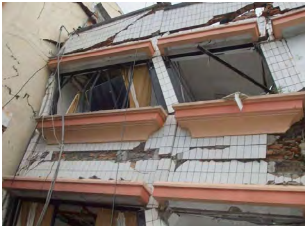
Figure 1.30. Plastic hinges at column ends
