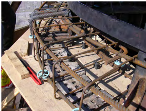
Figure 3.29. Reinforcing of the tower top beam
