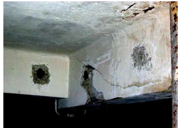
Figure 2.59. Inclined cracks at main beams
