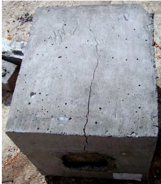
Figure 2.7. Fracture by longitudinal cracking at pull-off test
