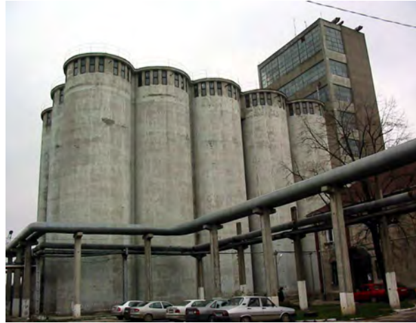
Figure 2.41. Reinforced concrete silos
