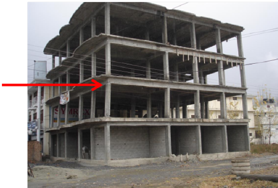
Figure 1.41. Permanent drift at the first floor of a reinforced concrete frame 4-storey structure under construction. Ground floor drift may have been prevented by the infill masonry walls
