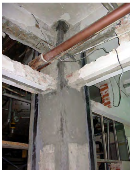
Figure 2.72. CFRP application for column longitudinal strips
