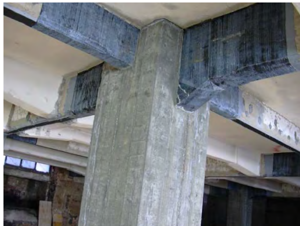
Figure 2.51. CFRP strengthening solution for beams
