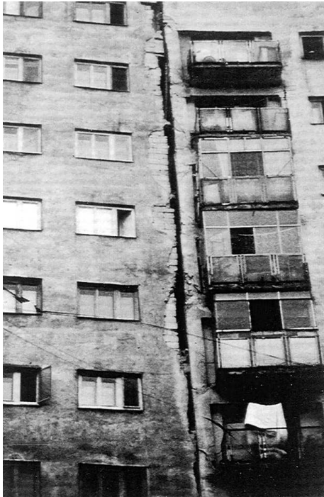
Figure 1.44. Bucharest, 1977: damage down the seismic gap line due to pounding [39]
