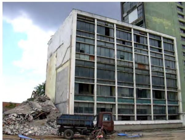
Figure 2.79. RC structure after demolition
