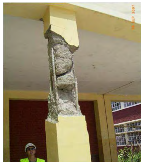
Figure 1.19. Column failure in shear due to insufficient shear reinforcement and low quality of concrete
