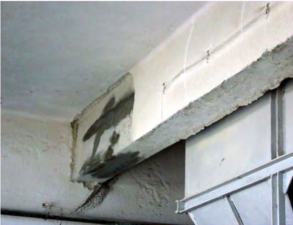
Figure 2.74. CFRP application for beams longitudinal strips
