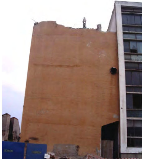
Figure 2.78. Partial demolition phase of RC structure
