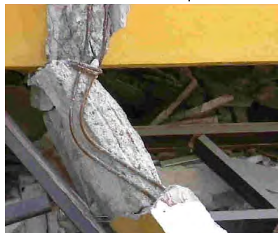
Figure 1.25. Slender columns, lack of bonding and absence of stirrups
