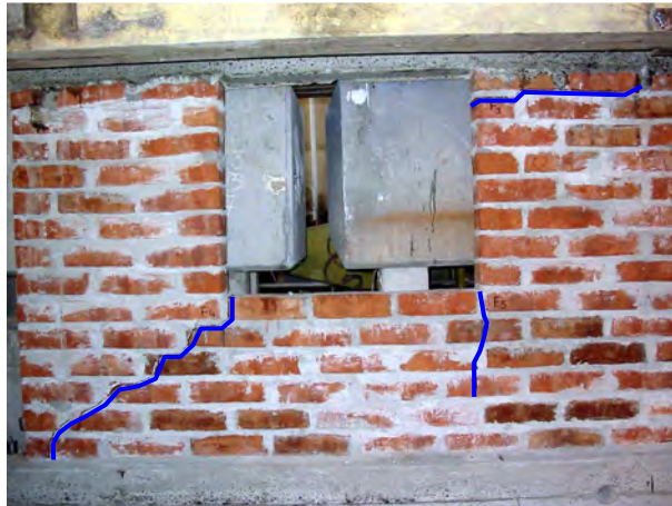
Figure 3.8. Un-strengthened masonry wall failure and crack pattern
