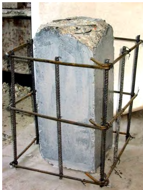
Figure 2.3. Using of bonding epoxy resin agent
