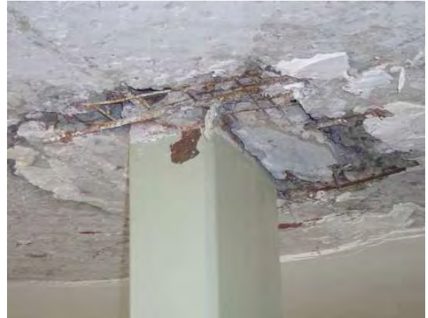
Figure 1.54. Punching of flats slab by column due to vertical seismic action
