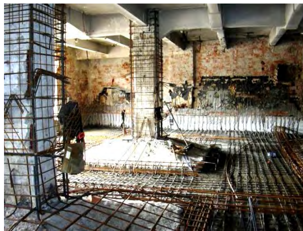
Figure 2.49. Reinforced concrete jacketing of columns and foundations
