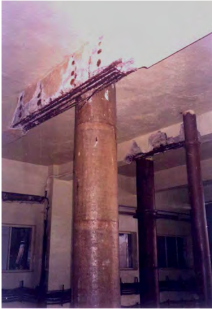
Figure 2.56. Damage of secondary beams
