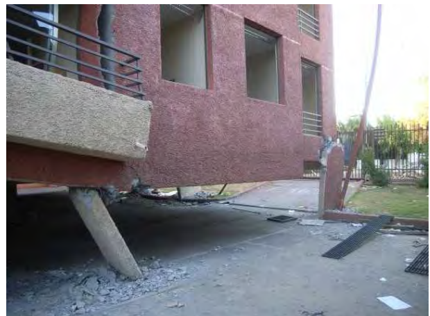
Figure 1.51. Soft ground storey collapse
