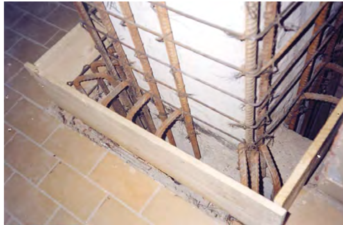
Figure 2.69. Reinforcement detailing at column-foundation joint (according to [88])
