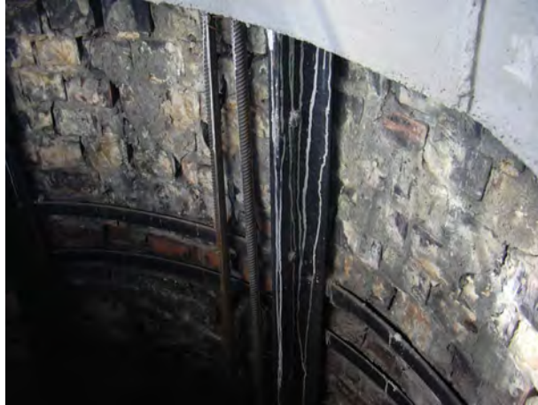
Figure 3.28. Vertical rebar and CFRP strips
