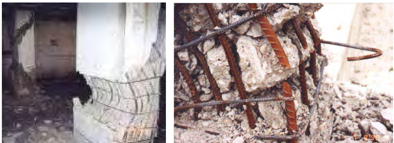
Figure 1.27. Plastic hinges in columns
