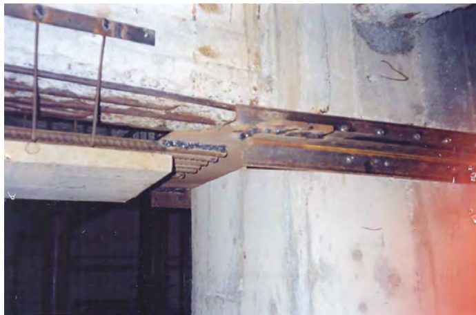
Figure 2.67. Anchorage detailing at beams end
