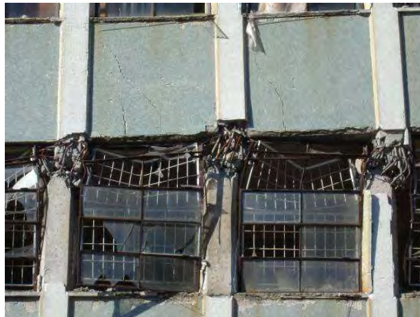
Figure 1.26. Plastic hinges in columns
