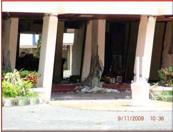
Figure 1.53. Soft ground storey collapse
