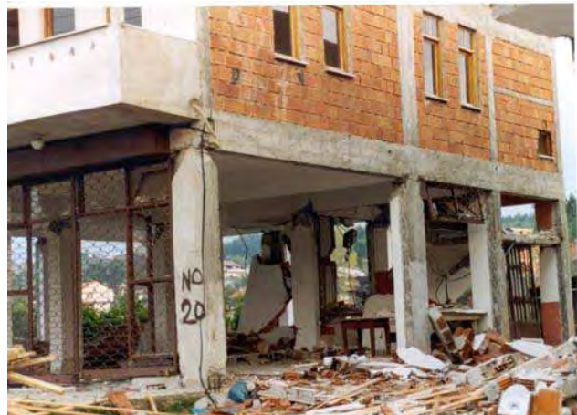
Figure 1.29. Hinges formed at bottom and top of columns
