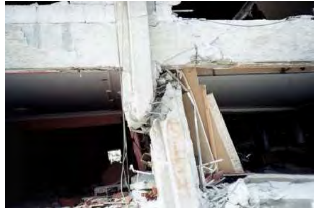
Figure 1.36. Shear failure at ground floor column
