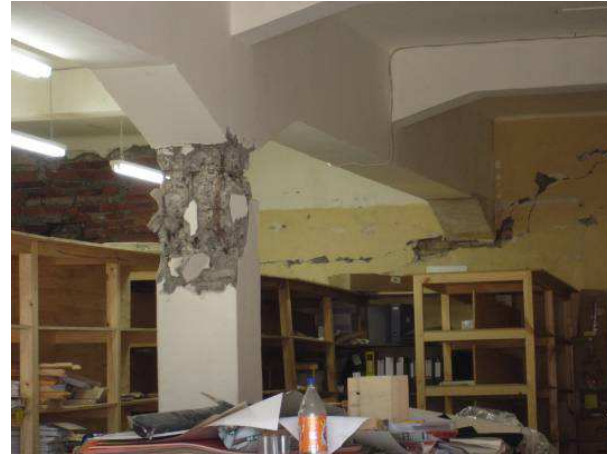
Figure 1.21. Insufficient shear reinforcement and low quality of concrete
