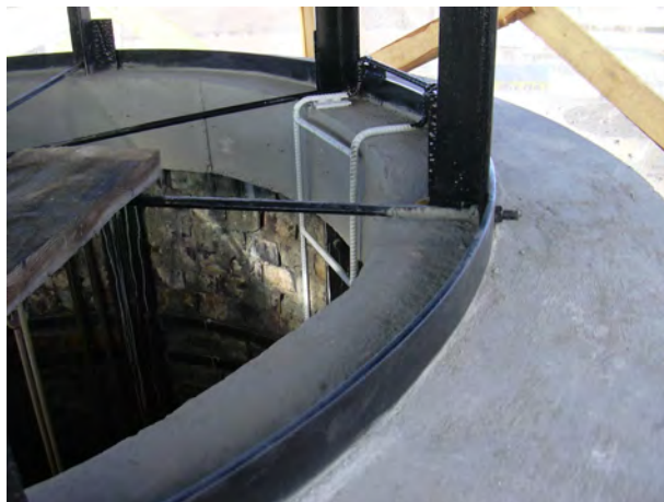
Figure 3.30. Reinforced concrete top beam
