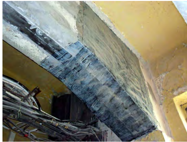
Figure 2.65. CFRP strengthening of main girder
