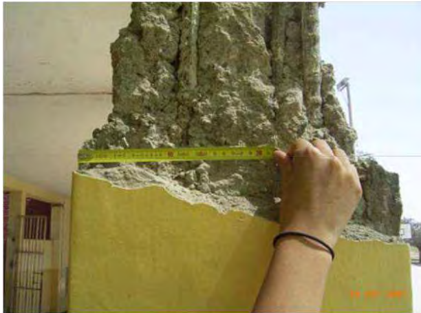
Figure 1.20. Excessive concrete cover, lowering design flexural capacity, and poor concrete quality
