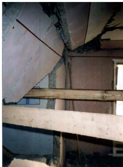
Figure 2.38. Fracture of reinforced concrete walls
