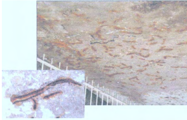
Figure 1.7. Corrosion of slab reinforcement
