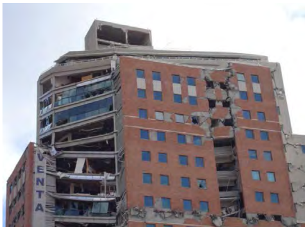
Figure 1.50. Collapse of different soft storeys with changed stiffness
