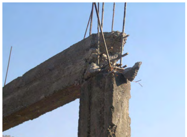
Figure 1.32. Roof columns failure
