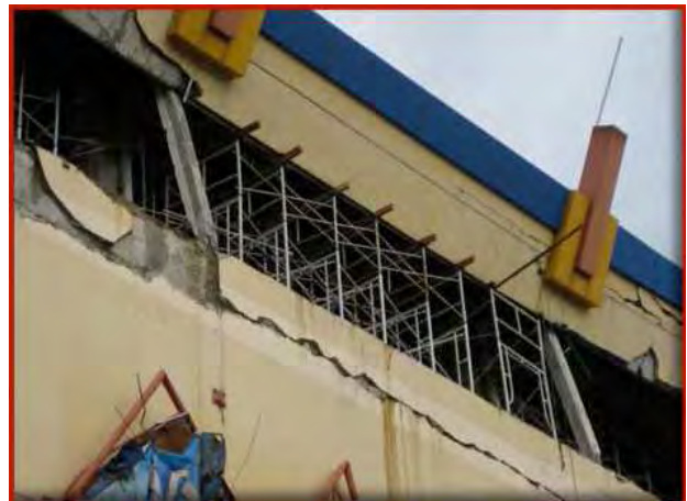
Figure 1.31. Roof columns failure
