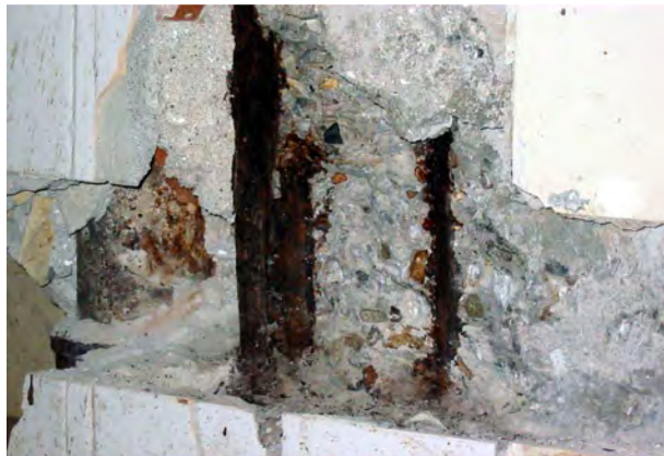
Figure 2.58. Damage of columns
