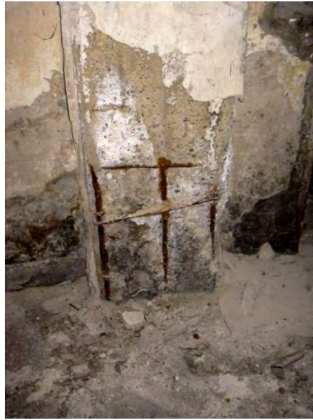
Figure 2.48. Damage of columns
