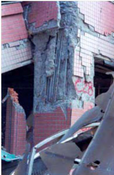
Figure 1.18. Lack of confinement at column head
