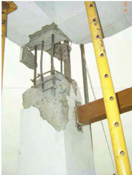
Figure 1.37. Failure of column at top end at the second storey, due to insufficient shear reinforcement and activation of a strong-beam-weak-column mechanism
