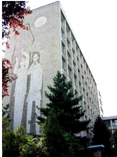
Figure 2.26. The Western University of Timisoara – Main Building
