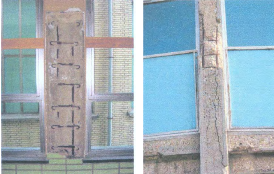
Figure 1.5. Corrosion of columns' reinforcement
