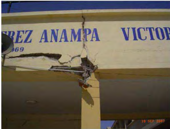
Figure 1.28. Column failure at top end: roof parapet activated a strong-beam-weak-column mechanism
