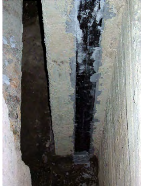
Figure 2.71. End anchorage of longitudinal CFRP strips for column
