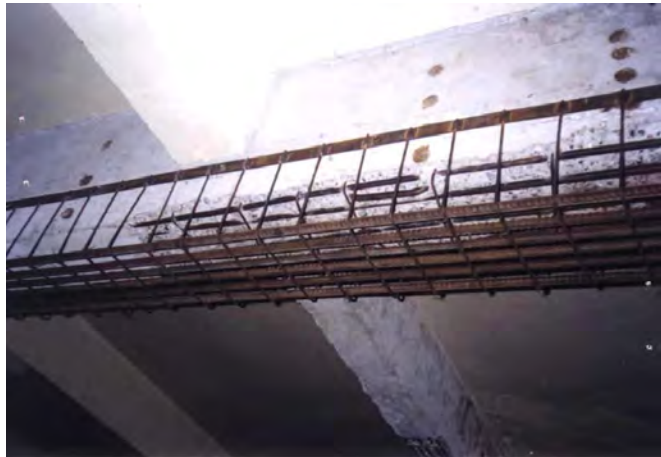
Figure 2.62. Reinforced concrete strengthening of main girder
