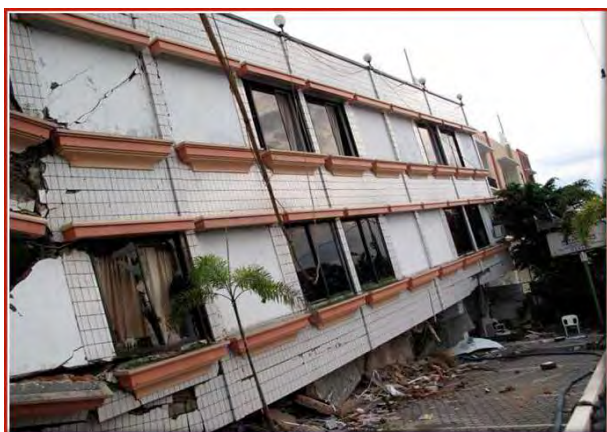
Figure 1.52. Soft ground storey collapse
