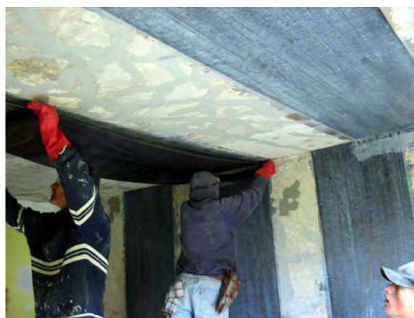
Figure 2.40. CFRP structural rehabilitation of walls and floors
