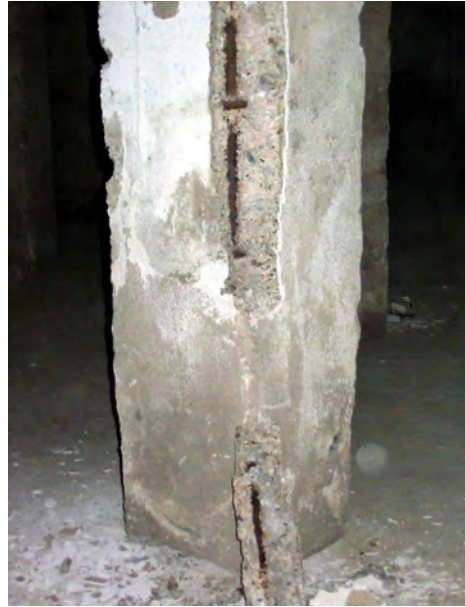
Figure 2.42. Reinforcement corrosion of discharge funnel
