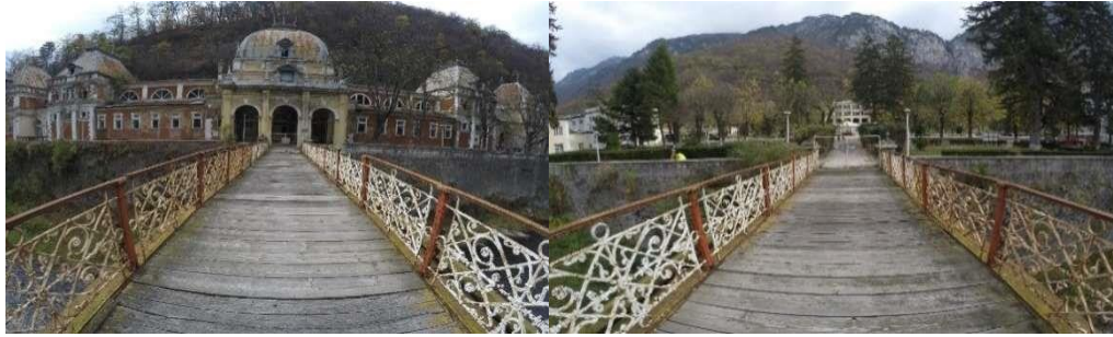
Fig 8. The current condition of the bridge
