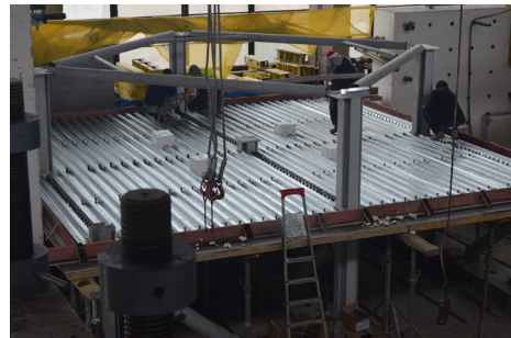
Fig. 6. Composite slab system during construction
